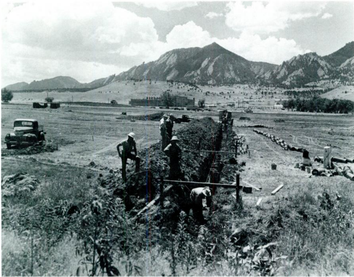
The site of Boulder Laboratories as it appeared on July 15, 1952, a few weeks after ground was broken for construction of the Radio Building. The tiled drain in foreground is located just to the north of the auditorium section of the Radio Building that was completed in the spring of 1954. In mid distance can be seen the Liquefier Building and the Camco Building, both constructed during 1951. Occupying the horizon at center is Bear Mountain, that provides a spectacular backdrop for the Boulder Laboratories in a southwesterly direction. Buildings of the National Center for Atmospheric Research now occupy the hilltop (known as Table Mesa) to the left and front of Bear Mountain.
