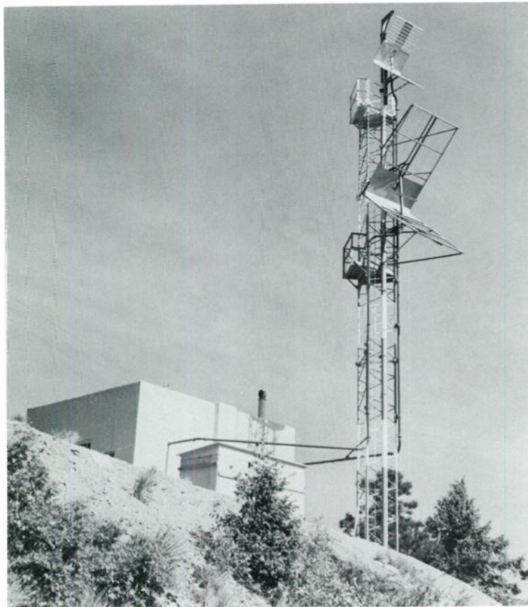
Closeup view of antenna tower at "base site," Cheyenne Mountain, showing details of the 92-MHz and 210.4-MHz (later modified to 236 MHz) transmitting antennas. The structure housing the transmitters is at the left.
