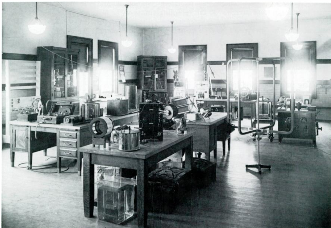
Wireless Laboratory, December 1915, located at north end of fourth floor, East Building. Many measurement instruments appear on the tables, including a standard capacitor and inductor, and Kolster receiver in center foreground. A two-coil direction finder is on the right.
