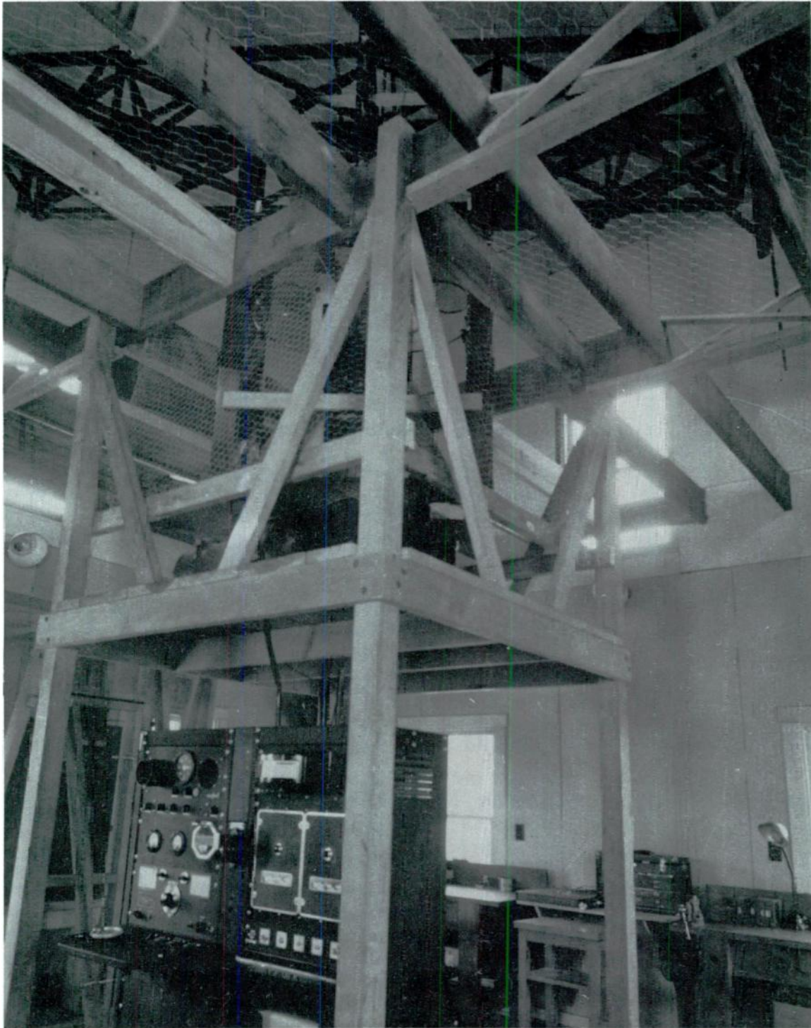
Interior of ground station at Beltsville, Md. field station for phase-variation method of observing wind speed and direction. The 22-MHz transmitter is at far left. Receiver and recorder at center. Above is the rotatable directional dipole array to determine wind direction. Balloon transmitter operated at 75.5 MHz.
