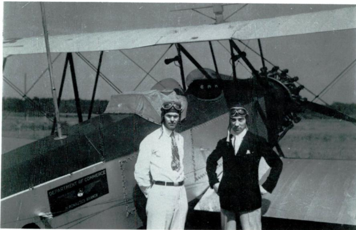
Department of Commerce pilot Marshall S. Boggs (left) and Colonel Clarence Young, Assistant Secretary of Commerce for Aeronautics, with Curtiss "Fledging" biplane used to make the historic first blind landing by radio navigation on September 5, 1931, at the College Park, Md. Airfield. Vertical antenna, located behind hooded cockpit, received signals from the runway localizing beam. Double horizontal antenna above upper wing received the glide-path signals.
