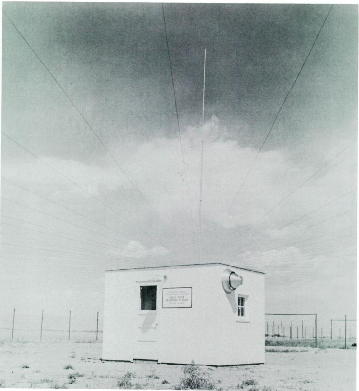
The NBS noise recording station located on Gunbarrel Hill northeast of Boulder, Colo. A whip antenna extends vertically above the center of an elevated ground plane consisting of wires radiating horizontally from the base of the antenna. Such a ground plane stabilizes the antenna impedance. This station was one of 16 scattered over the World for the IGY noise program of 1957-1958, 5 of the stations being operated by the NBS.
