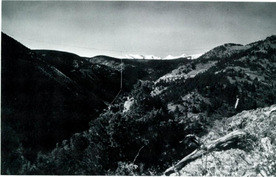
View to west at Sunset in Four-mile Canyon, northwest of Boulder, with Continental Divide in distance. Across canyon was stretched a cable that served as the antenna for experimental transmission of standard frequency at 20 kHz. Scheduled operation of station WWVL began on April 5, 1960. Accuracy of frequency measurement at several thousand miles distance was increased by one-thousand-fold over broadcasts from WWV. In 1963 operation of WWVL began at the Ft. Collins, Colo. site.
