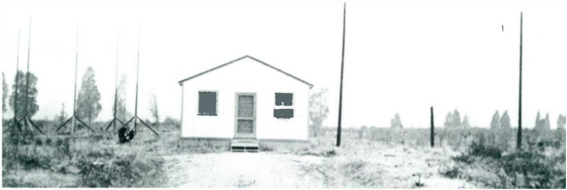
The Warning Service Building was one of four buildings used by the CRPL in its 16-year operation (beginning in 1949) of the Fort Belvoir field station south of Washington, D.C. The antenna structure at left of building was for the direction finder, the antenna at right was for field-intensity measurements of transatlantic circuits.
