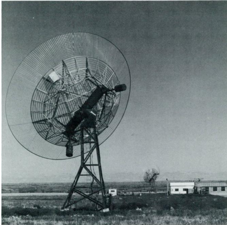
Two 40-ft diameter paraboloidal antennas at the Table Mountain field site, north of Boulder. These two “dishes” are mounted at the ends of a 475-m base line to form a Ryle-type radio interferometer for studying signals emitted by non-terrestrial radio sources, especially from Cygnus-A and Cassiopeia-A. The project mechanic, standing to the right of the nearby support structure, indicates the large size of the steerable antennas.
