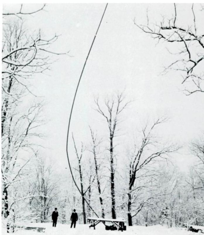
Antenna mast, buckled by a snowstorm of March 1914, was located to the east of the recently constructed East Building that housed the Bureau's radio laboratory. (Original print shows the arrays of guy wires "supporting" this mast.) It is the only known picture of a radio antenna associated with this laboratory.
