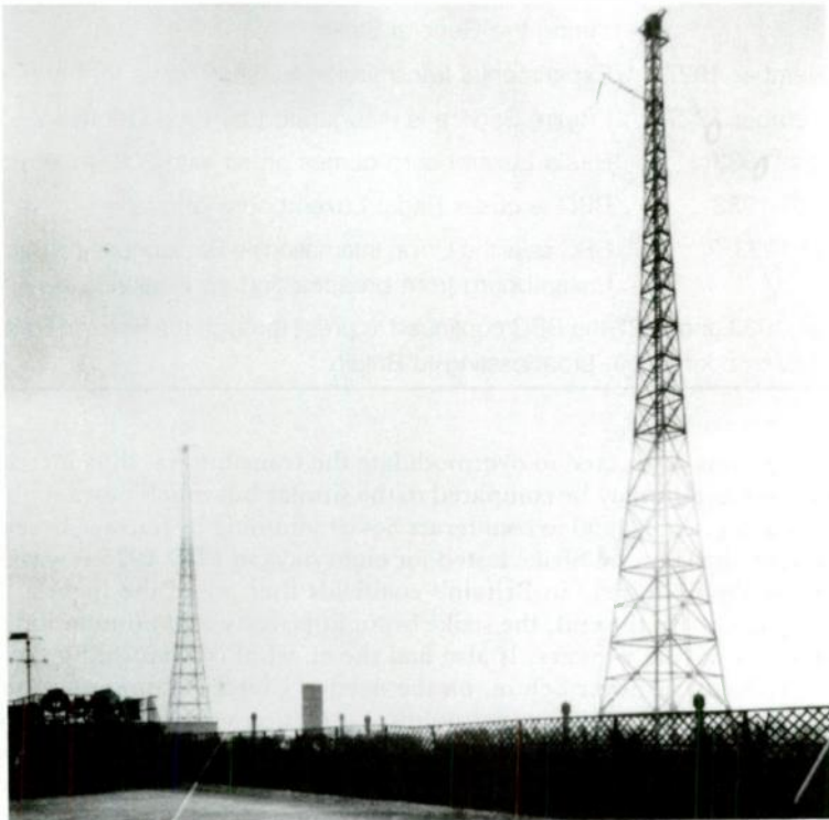
Figure 5.1 Aerial system for 2LO BBC, 1927, on roof of Selfridges Department Store, London
