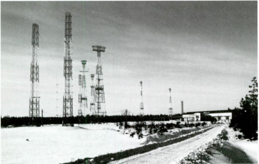
Figure 22.2 The Pori SW station (Finnish Broadcasting Company) under snow
