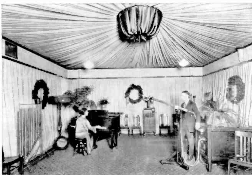
KDKA's first real studio, 1922. Note the draped ceilings and walls which at the time were the approved method of obtaining the proper acoustic effects. (Courtesy Westinghouse Electric Corporation)
