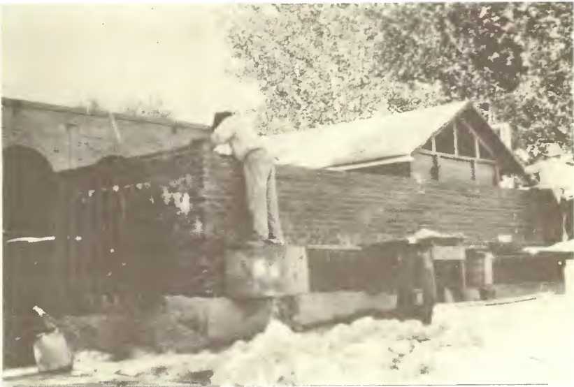
New transmitter house being constructed around the old Radio Shack, 1927. Later, the wooden structure was removed piece by piece through the door of the new house. Broadcasting service was interrupted only once during the transition.
