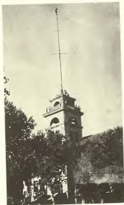
Dean Goddard standing on the tower of the Engineering Building to assist Robert W. Stewart (at top of mast) in attaching supporting cables to the 120-foot aerial. (R. W. Stewart photo)
