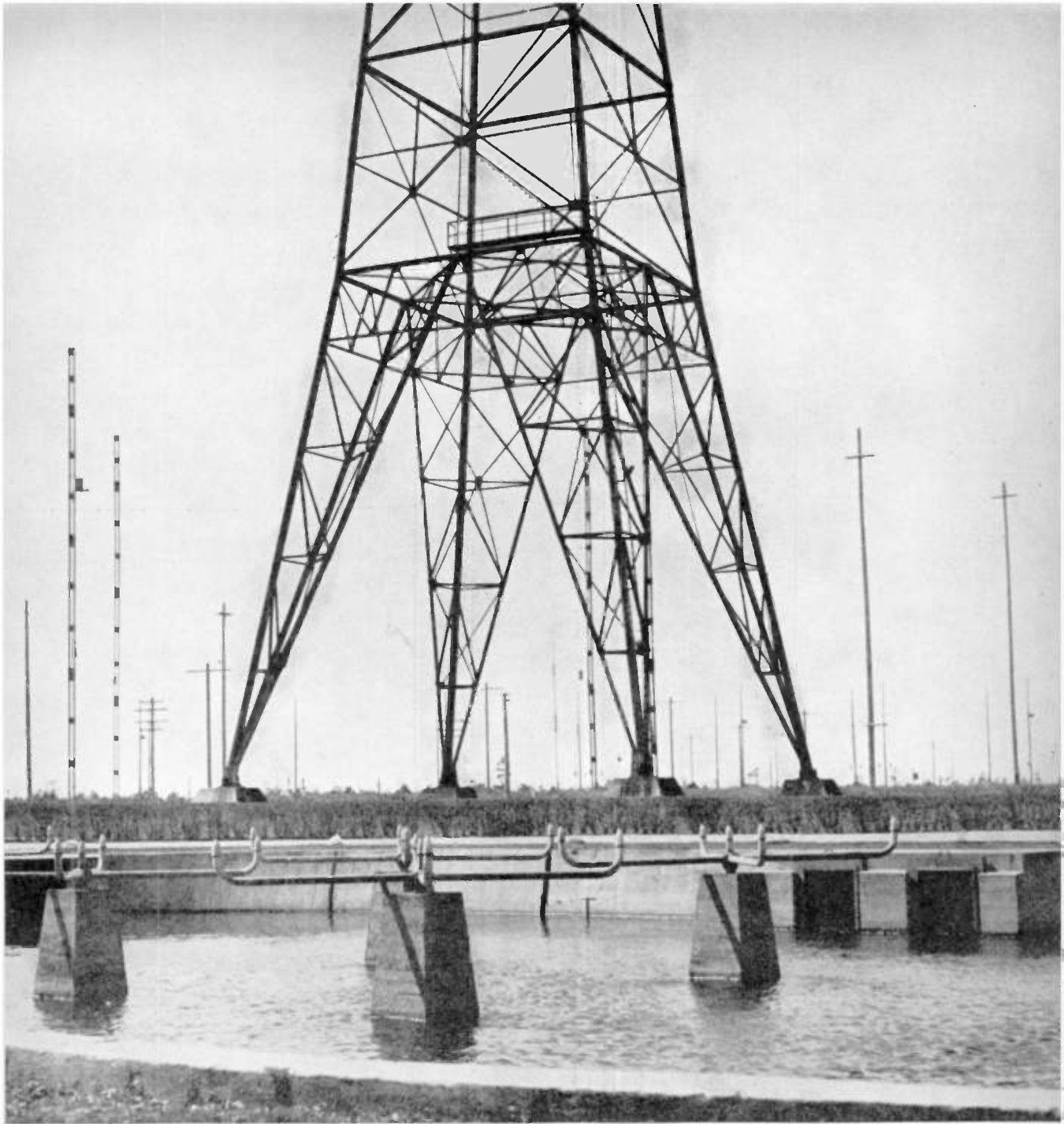
A "cooling pond" lowers the temperature of water used to cool the tubes and machinery in the high-power radio transmitters
