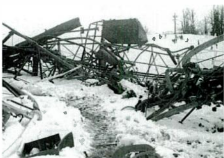
Sections of KOIN-TV towers in mangled heap following their collapse on February 28, 1971
