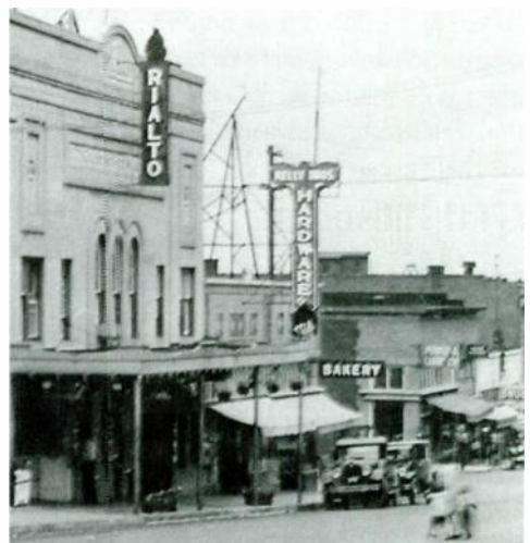
Rialto Theatre at the time of KFHB's operation with antenna towers visible on adjacent roof
