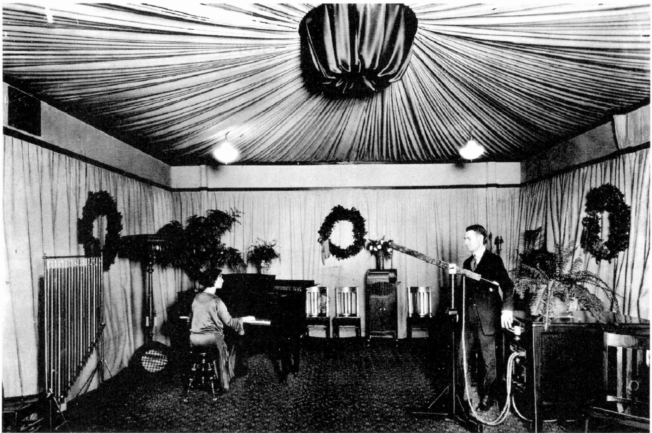
Acoustics became important in early broadcasts, forcing stations to drape their studios, like this early KDKA studio in Pittsburgh.
