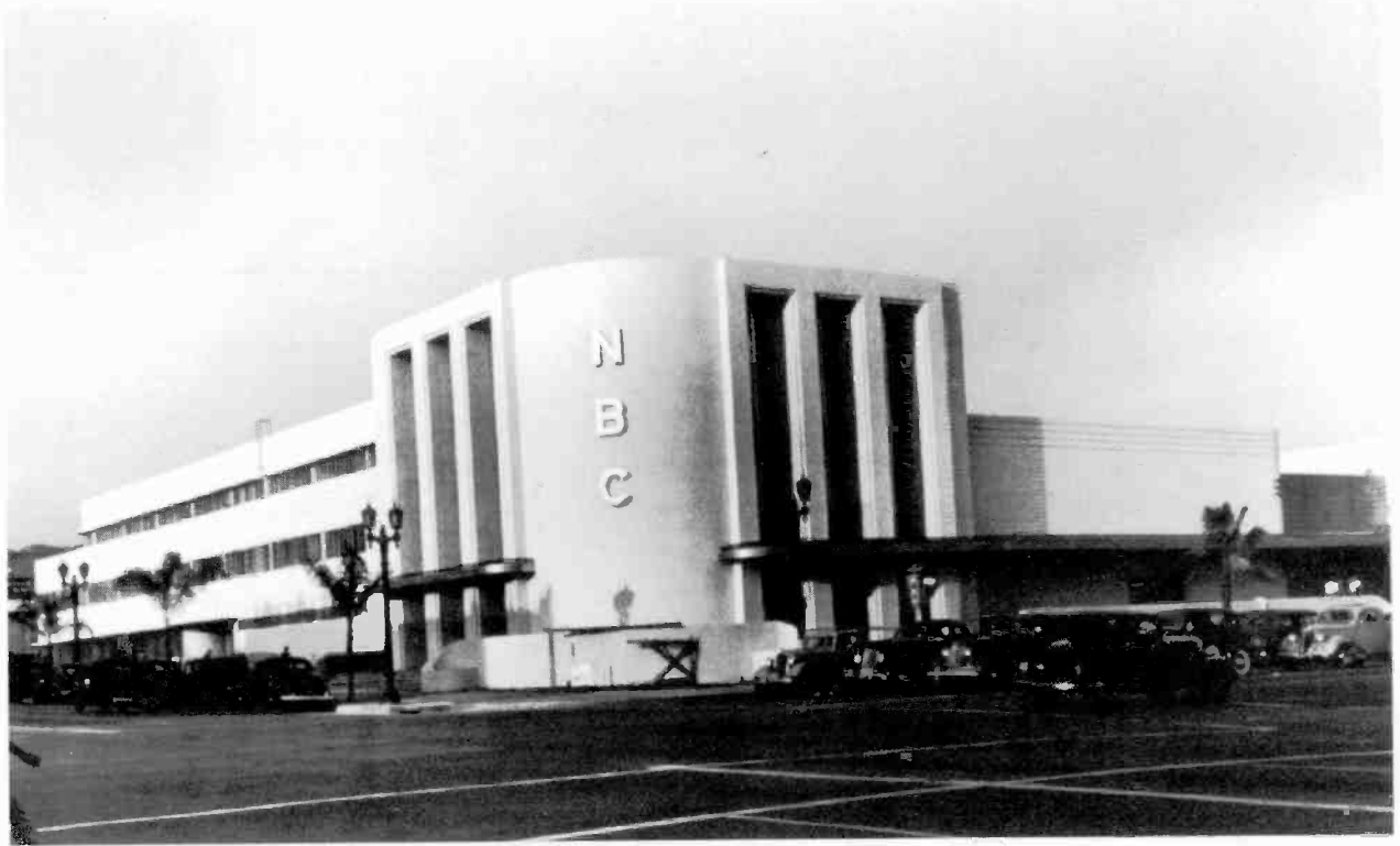
Radio was booming and the networks were making more money than ever imagined, resulting in palaces for network operations. This was the new NBC facility in Hollywood.
