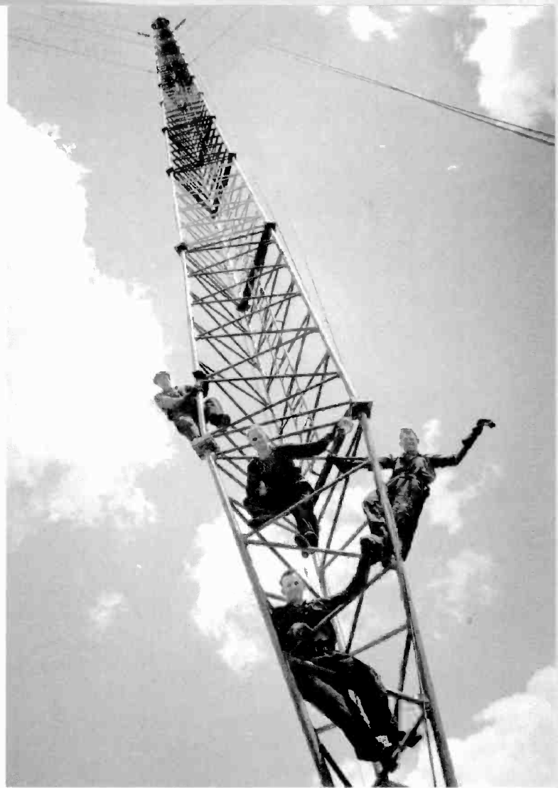
Riggers climbed the KDKA tower daily during its construction. The innovative free-standing tower was 718 feet tall and built of 60 tons of metal.
