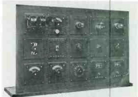
Front view of 15 Panel "Type 15" De Forest Unit Receiver Set" containing 15 tubes with wave length range of 100 to 4,000 meters, 3 trays of 100 and 500 ohm resistors, and a 400 ohm amplifier. The most efficient receiver mounting apparatus ever put on a radio station.
