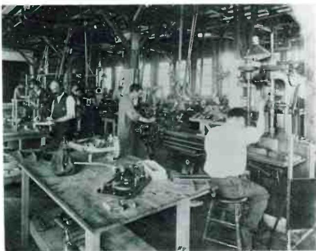
Machining rotary spark gaps, 1917.
