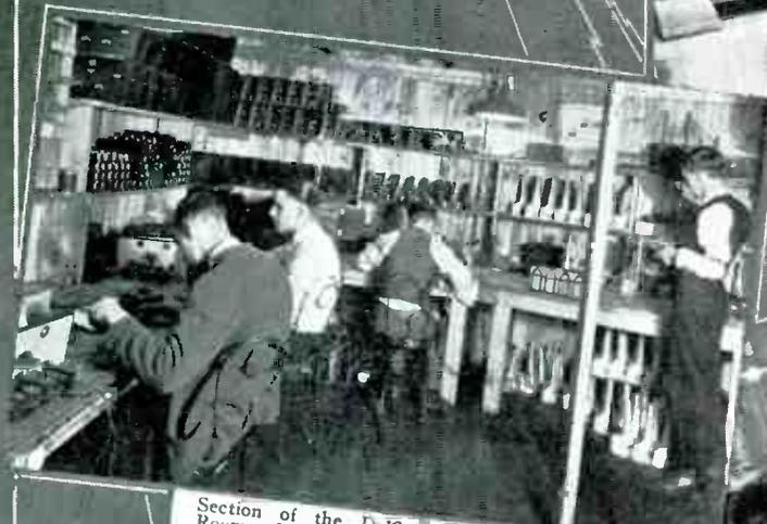
A section of the Trirdyn Room, showing lines of workers engaged in the wiring of these Radiophones. On the left, note the inspector testing.
