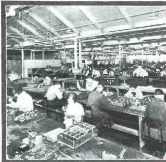
Above we see a big assembly room, where the units of parts from the various stamping, winding, and other machines are brought together, and united into complete apparatus by deft operators. Long stretches of benches can be seen in well-lighted rooms, where one operation follows another in quick succession. The suitable routing of assembly work is one of the greatest factors in high-quality and low-cost manufacture today.
