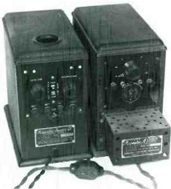
In the 1924-27 period, before AC sets were fully established, B-battery eliminators rang up more than \$30 million in sales, the most popular model being the Majestic Super-B. A-battery eliminators were less successful, as no really good rectifier was available for the high currents needed (1½ amperes for a six-tube radio).
