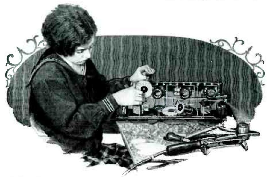
The Basket-Woven Inductance Coil Follows the Antenna and Tickler Coils into Place as the Growing Set Flits down the Long Assembly Table
