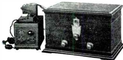
Model 66AC—Six tube AC operated two unit model—Receiver and A & B power—complete with B eliminator tube, but less AC tubes. . . . \$155.00
