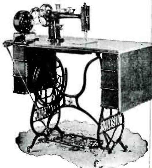
THE KENT ALTERNATING SEWING MACHINE MOTOR.
