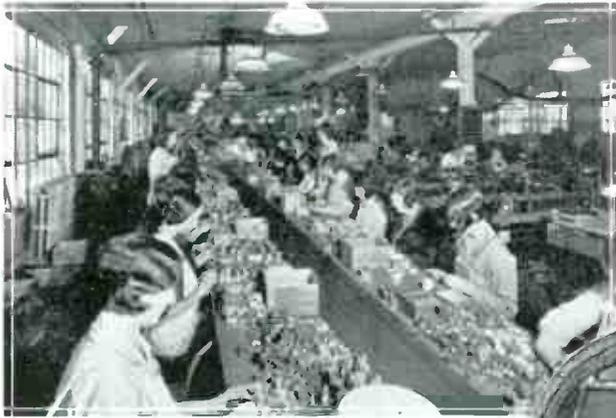
**ARMATURE ASSEMBLY.** The young women in the picture are assembling the most important part of the Dynacone, the armature. The armature oscillates between the poles of two powerful electro-magnets and the length of the oscillation determines the depth of tone.
