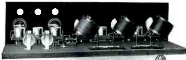
The rear view of the five tube home-made "Neutrodyne" receiving set. Audio frequency amplifying transformers on this set are both placed to the rear of the triple tube socket.
