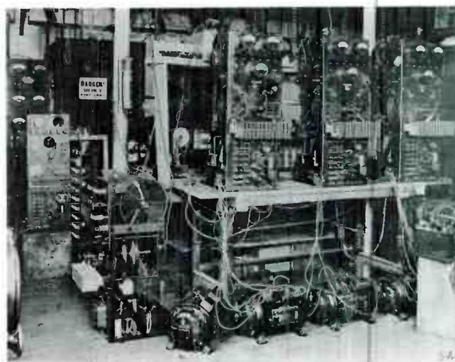
Testing quenched-gap transmitters, about 1919.
