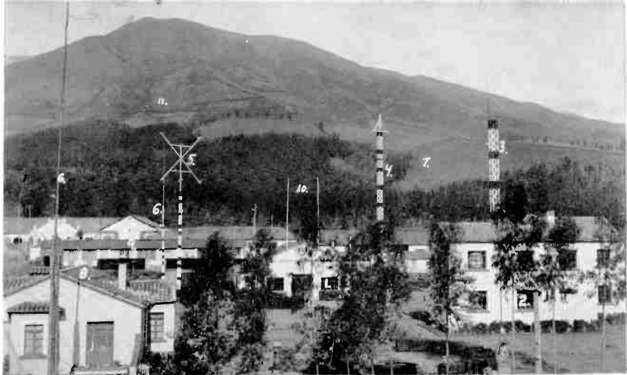
HCJB GROUNDS: 1. Transmitter Building, 2. Studio and Office Building, 3. 24-meter Tower, 4. 31-meter Tower, 5. 19-meter Tower, 6. Long-wave (308) Antenna, 7. 49-meter Antenna, 8. Co-directors' Home, 9. Bodega Apartments, 10. Flagpoles, 11. Mt. Pichincha.
