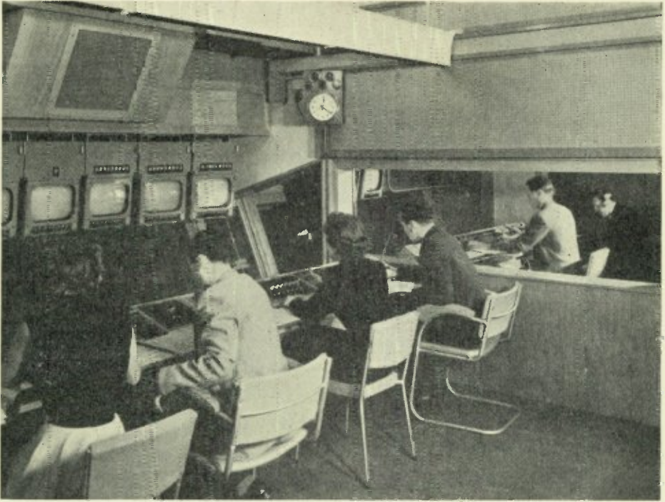
A B.B.C. control room, with vision in front and sound behind the partition. Notice the 'monitoring' T.V. screens showing what is happening in the studio.
