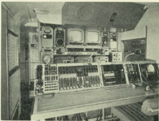
Interior view of a mobile control van for outside broad- casts
