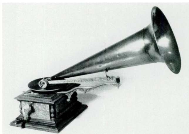
"Grand Opera," 1901-04. Until the addition of the "Royal Grand" in 1905, the Grand Opera represented the top of the Zon-O-Phone line. The fancy oak case has a beveled glass window on either the front or the back. This one is on the back and therefore cannot be seen in the photo. The single-spring motor could play five 10" records. The turntable was still 9" and the horn was 30". The Grand Opera cost $45.00 in 1904. (Peter Dilg collection)
