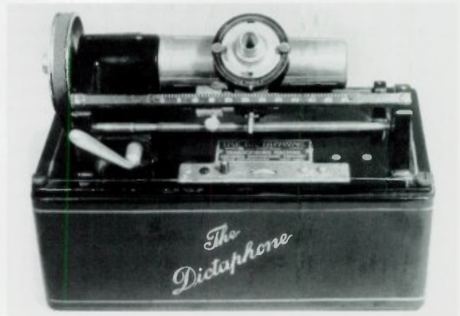
The Dictaphone, c. 1915. The Dictaphone shown here is also an electric machine. The reproducer is a variation of the "Lyric" and is not capable of recording. This machine remained, with minor variations, the basic dictation unit sold by Columbia until the early 1950's. (Author's collection)
