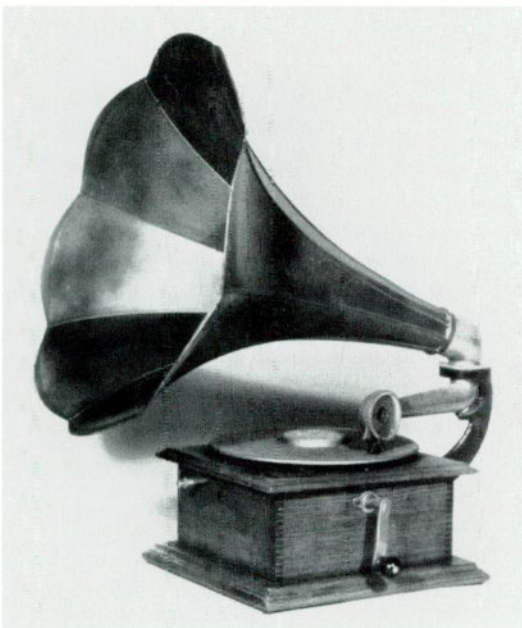
Aretino, 1909-14. After Columbia started to manufacture the Aretino, the machine received a characteristic Columbia motor with a combination on/off/speed control projecting through the front of the case, and a typical Columbia tone-arm. (Ernie Bennett collection)
