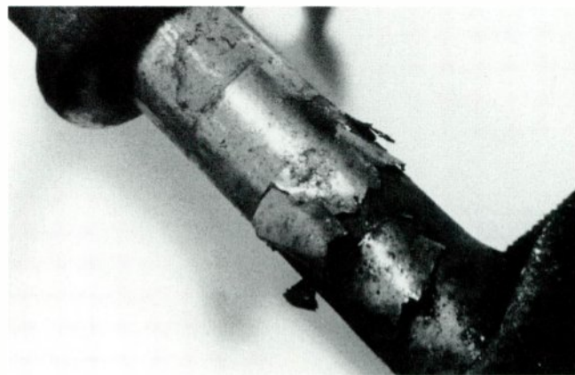
The peeling plating on this crane is due to improper preparation of the plating surface—and probably an improper nickel bath.
