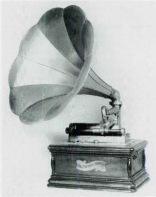
Model C "Universal," 1897-1905. The Universal was designed as an office machine, but was recommended for phonograph exhibitions because of its powerful triple-spring motor, which Columbia claimed could run for an entire hour at 120 rpm! That's the equivalent of 30 two-minute cylinders—quite a lot for most triple-spring machines. The cabinet is "black oak" and has a flip-down front for motor access. An electric version was also produced. The Universal sold for $50.00. (Ernie Bennett collection)
