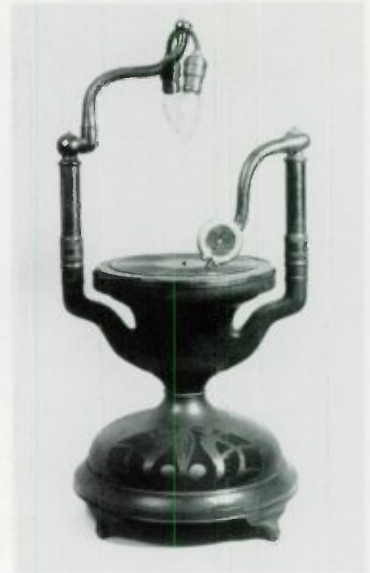
The Fairy Phonograph Lamp, c. 1918-23. The Fairy Phonograph Lamp was produced for a number of years by the Endless-Graph Co. of Chicago. Volume controls and on/off switches are hidden in the side columns. Although the lamp is made of copper and many collectors polish them up, the copper was originally painted to resemble dark green oxidation. This model has a 12" turntable, but a 10" model also exists. The lampshade is a good copy of the original, but is a few inches taller than it should be. Right view shows the machine in use. The shade has been removed for the sake of clarity. (Author's collection)
