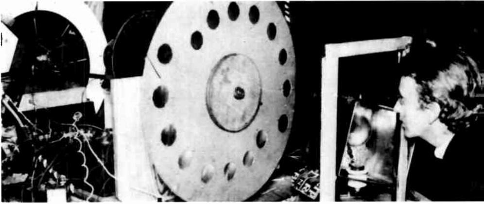
Between 1923 and 1925 John Logie Baird, an eccentric, sickly Scotsman with no scientific training whatsoever, developed a working television system based on the Nipkow disk. His only previous success had been the “Baird Undersock.”
