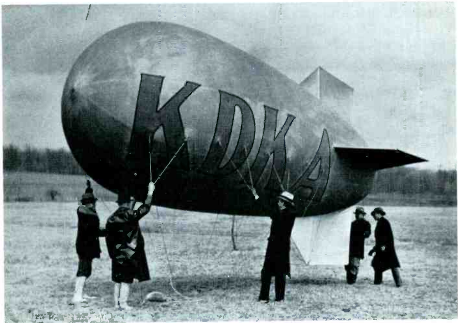
KDKA experiments with balloon antenna.
