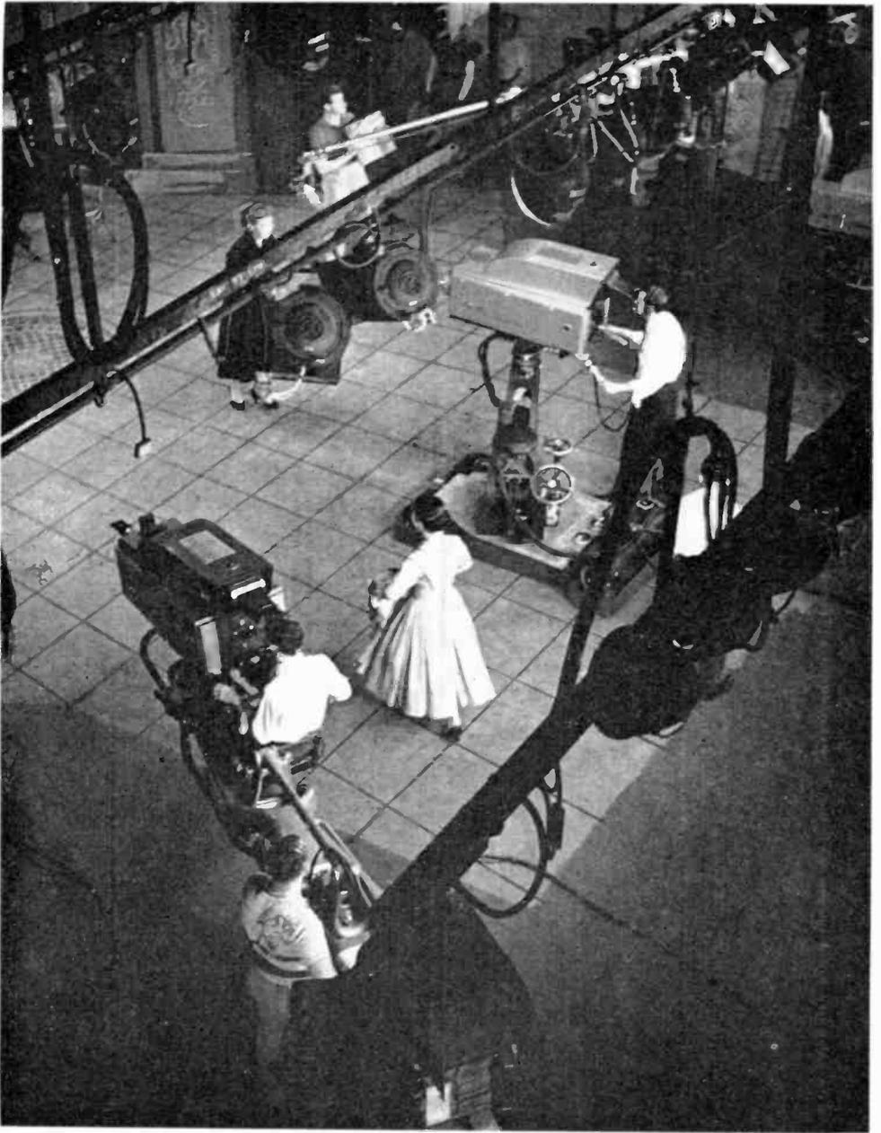
*Fig. 11 – Colonial Theater staging area. Taken from the balcony, this photograph shows part of the opening scene of the April, 1953, demonstrations. Crane and dolly cameras, microphone boom, and foreground lights are also shown.*
