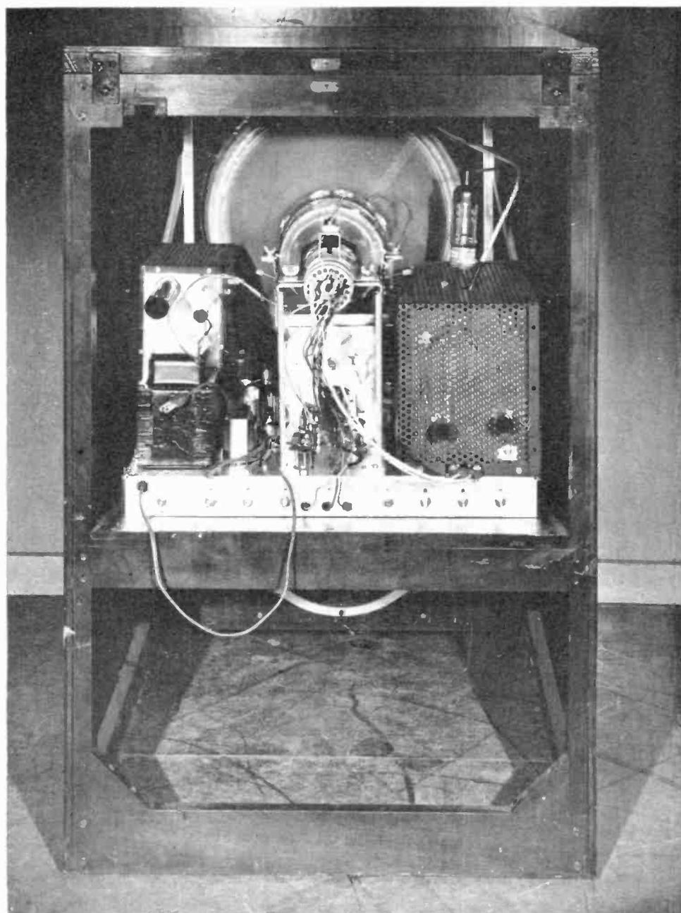
*Fig. 10 – 16-inch Tricolor Kinescope Receiver Model No. 3*
