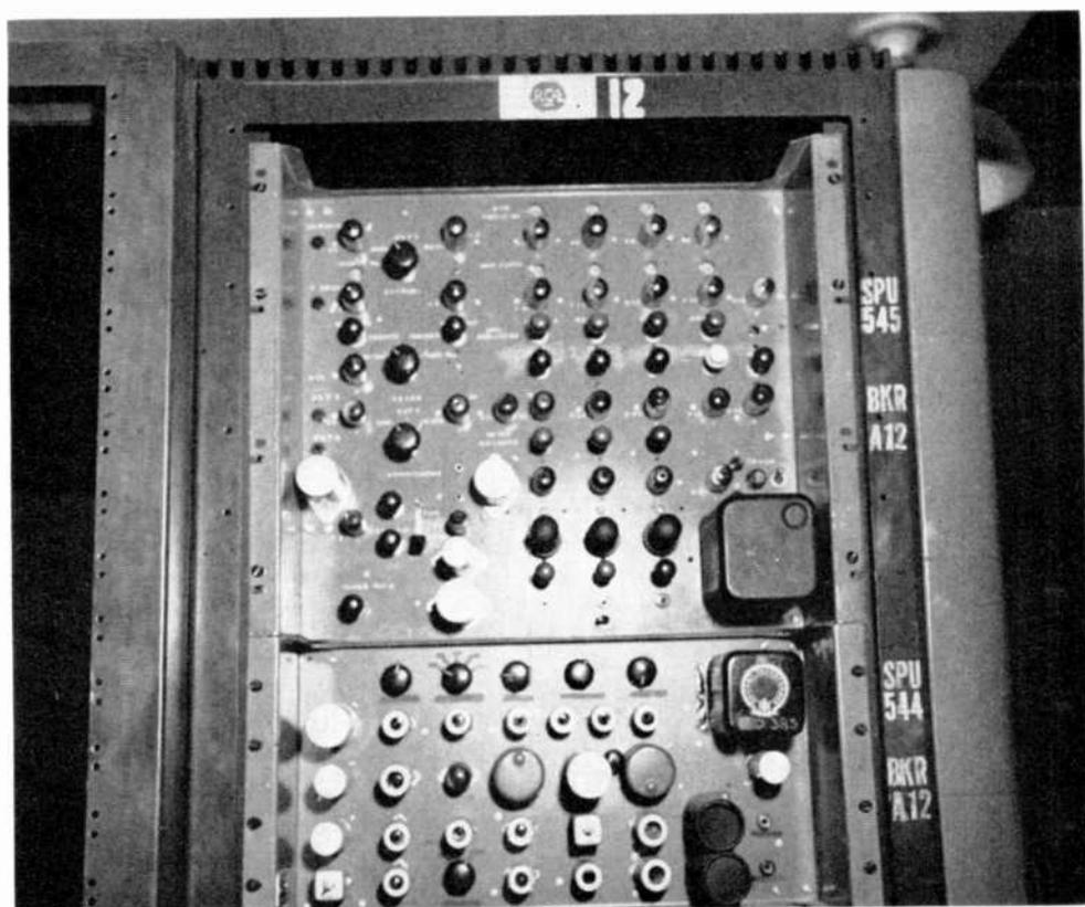
*Fig. 43 — Color-bar generator (upper chassis).*
