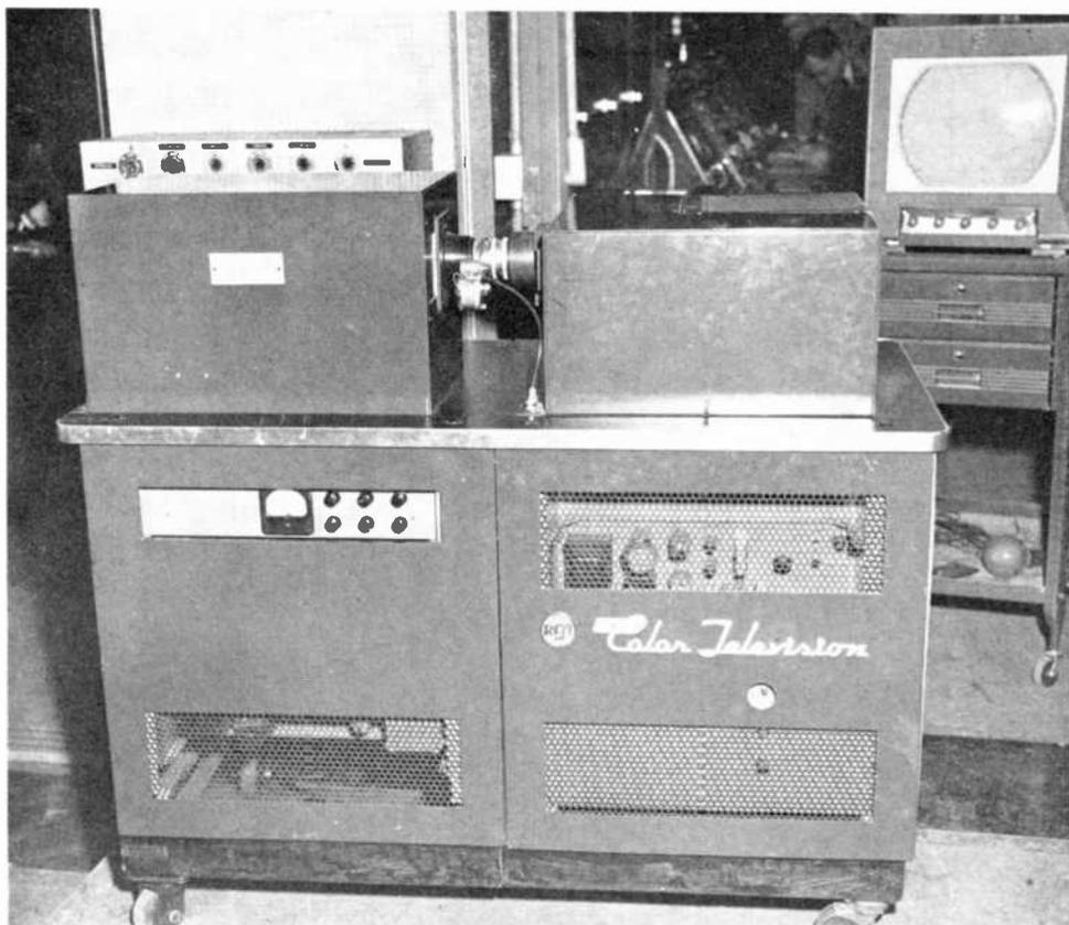
*Fig. 28 — Flying-spot scanner.*
