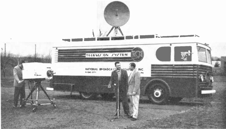
Fig. 53 — Remote pickup unit for RCA color television.
