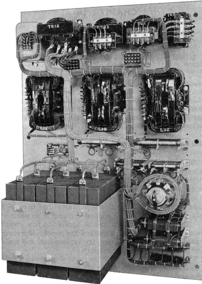
**Fig. 14-1. Magnetic Amplifier Type Voltage Regulator for 200 KVA Generator Using Three-Phase Metallic Rectifiers. (Courtesy of Vickers, Inc.)**
