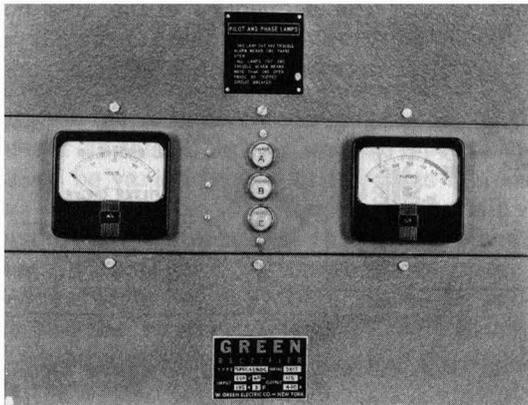
**Fig. 10-3. Front View of Supervisory Controls on Rectifier System Shown in Figs. 10-1 and 10-2. (Courtesy of W. Green Electric Company.)**
