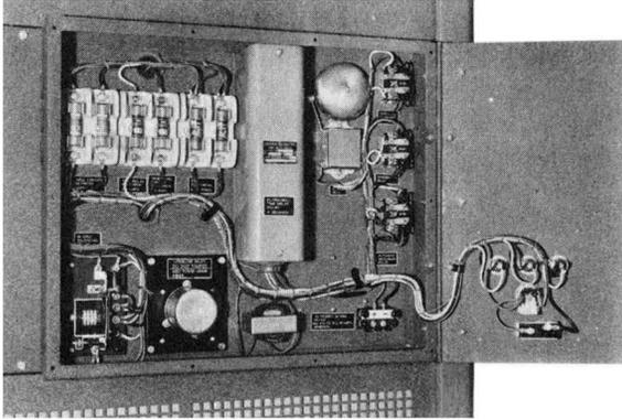
**Fig. 10-4. Interior View of Supervisory and Automatic Controls On Rectifier System Shown in Figs. 10-1 and 10-2. (Courtesy of W. Green Electric Company.)**
