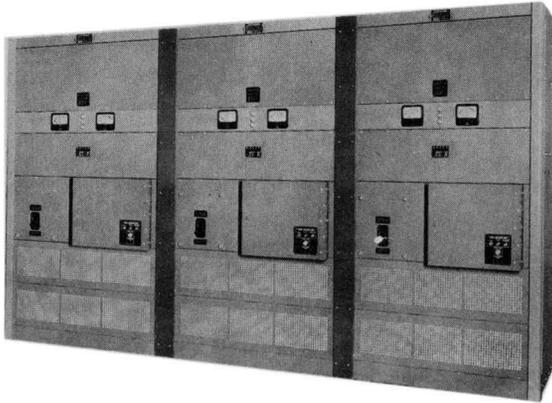
**Fig. 10-2. A Selenium Power Rectifier System Using Three of the Units Shown in Fig. 10-1. (Courtesy of W. Green Electric Company.)**
