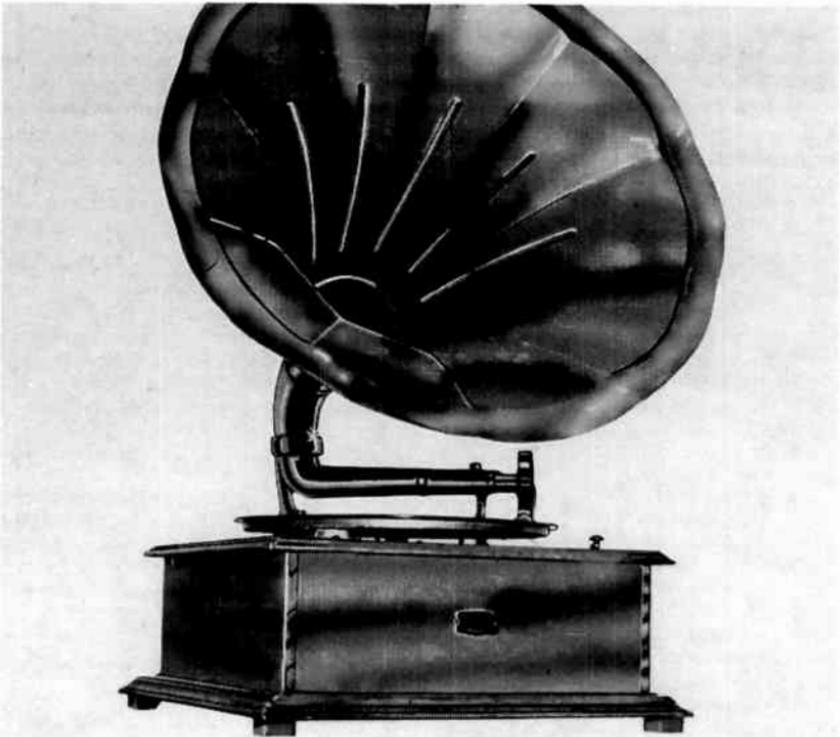
*Fig. 14-7. A Pathe spring-wound phonograph using a diaphragm type reproducer responding to vertically cut records.*
