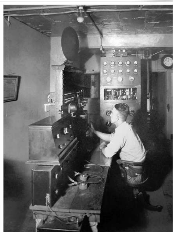
KFNF Transmitter Room, 1927.
