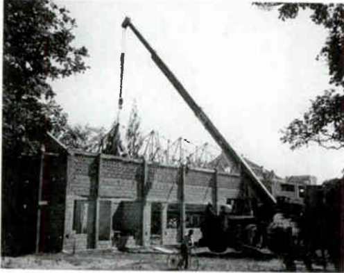
The borrowed crane hoists the steel trusses into place (1983)
