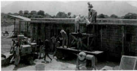
1959 construction of the transmitter building
