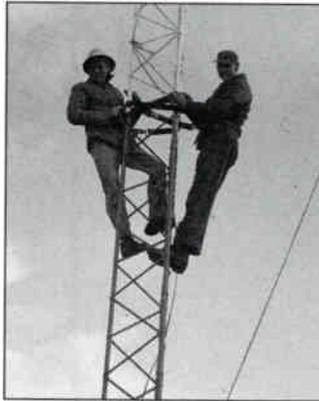
**Bill Hartman and Ralph Fondell assembled the 250-foot tower in 10-foot sections.**
