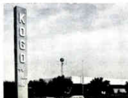
From land and air, the KOGO tower is a familiar sight.
