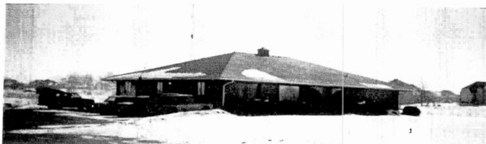
Rockford's WNTA (WKKN) and WKMQ on Reid Farm Road.
