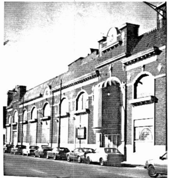
Fred Mann's Rainbow Gardens, 4836 N. Clark Street. This building one had two towers on the roof and is now used as a skating rink.
