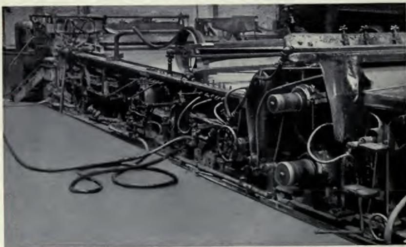
WHERE wood pulp is turned into Tribune newsprint. Wood pulp greatly diluted with water flows on a wire screen at the left of this picture. When it reaches the right end the water has been drained out, the fibres matted; it has become a sheet of wet paper—ready to pass through the series of rolls, blankets and driers, which finish the process.
