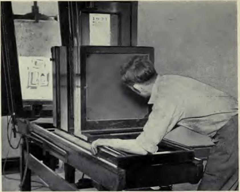
*The first step in making an engraving is shown above—photographing the original. Below, the etcher has just taken the zinc plate out of the acid bath after a "bite."*
