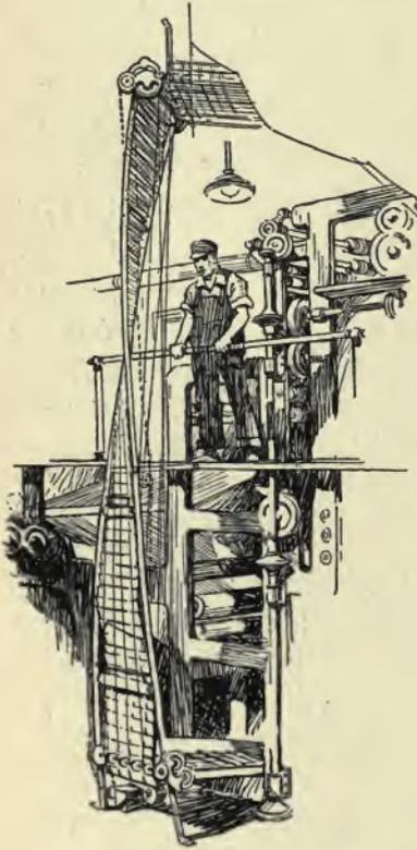
Each conveyor consists of spiral-wound, wire spring cables facing each other and running over pulleys. The pressure of these cables against each other holds the papers firmly between them and carries them swiftly upward.
