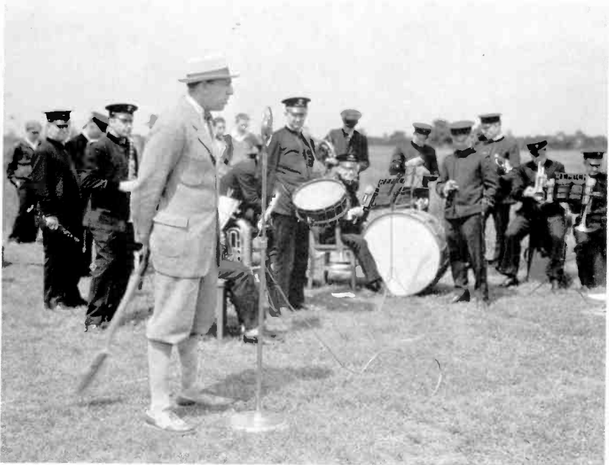
Crosley, in knickers, at Mason, Ohio, groundbreaking, 1928 Cincinnati Historical Society
