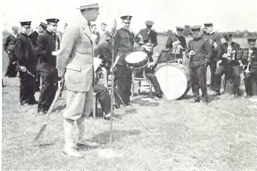
Crosley, in knickers, at Mason, Ohio, groundbreaking, 1928
