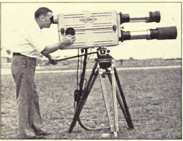
Courtesy National Broadcasting Company FIG. 29a—Camera in field operation, with use of telephoto lenses.
