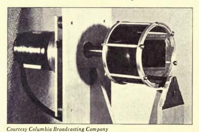
FIG. 59—Color Television. Filter drum and mirror used in the Columbia Broadcasting Company system.
