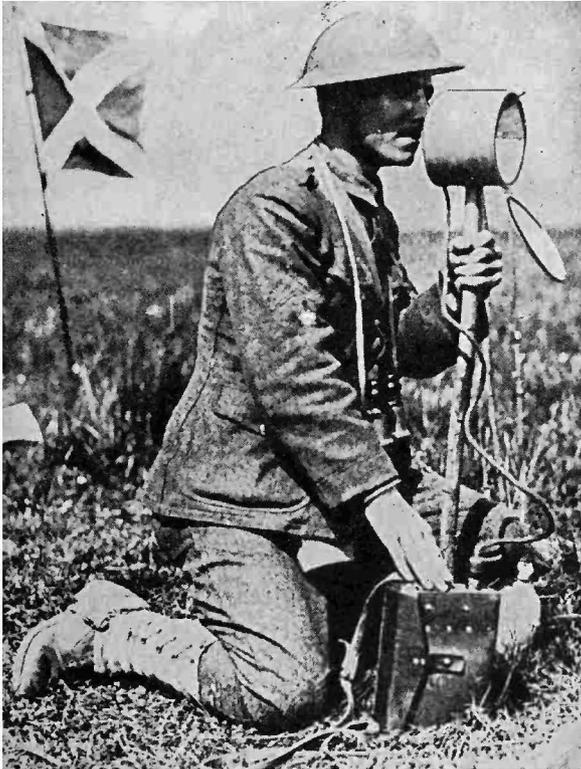
FIG. 1-5.—Signaling by means of a heliograph. (From the *Special U.S. Army Signal Corps Issue of Radio News*, photograph by U.S. Army Signal Corps.)
