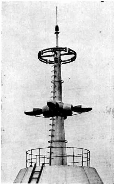
FIG. 169.—Radiator system designed by Lindenblad for station W2XBS, the National Broadcasting Company's transmitter atop the Empire State Building in New York City. The top structure is the folded dipole used for sound transmission, the lower the constant-impedance turnstile structure for the picture signal.
