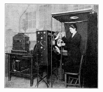
John Geloso and His Compact Television Transmitter. His Left Hand Is Resting on One of the Photoelectric Cells That Pick Up the Light Reflected from the Surface of the Image.
