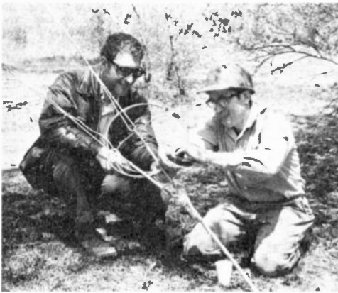
Fig. 14-12 — A guy cable is used to assure the turnbuckles remain in place after they are tightened. This procedure is an absolute requirement for a guyed tower system. (Photo by K1THQ)
