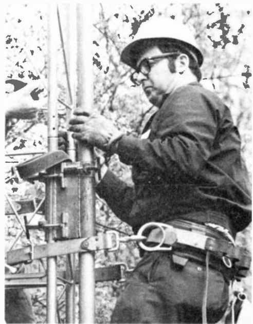
Fig. 14-13 — A good-quality safety belt is a requirement for working on a tower. The belt should contain large steel loops for the strap snap. Leather loops at the rear of the belt are handy for holding tools. (Photo by K1THQ)
