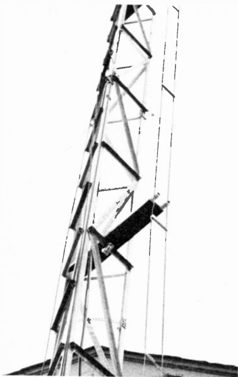
Fig. 13-12 — A board fitted with standoff insulators and clamped to the tower with U bolts keeps open-wire line suitably spaced from a tower. (W4NML.)
