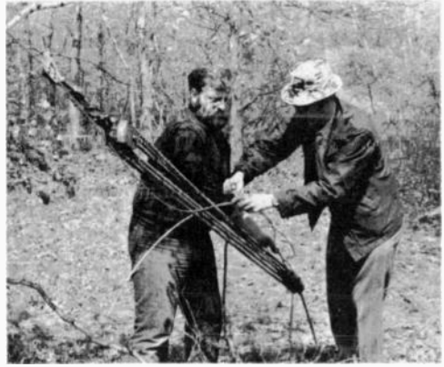
Fig. 14-11 — Proper tension can be placed on the guy wires with the aid of a block-and-tackle system. (Photo by K1THQ)
