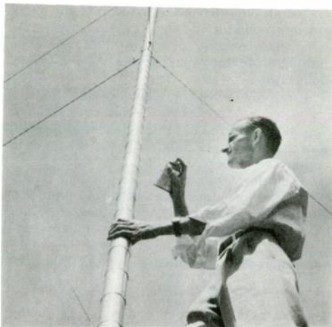
The "Budget 7-Mc. Vertical Antenna" described in November, 1955, was a tongue-in-cheek but nevertheless practical description of a beer-can vertical. The caption to this illustration read, "Here W2JTJ is touching up a spot on his antenna he missed with the aluminum paint the first time around. A lot of thought and libation went into the construction of this vertical."
