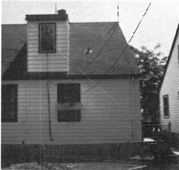
The house serves as both an anchor point for the fold-over pulley and a supporting structure for the lower half of the tower.
