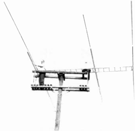
Fig. 8-14—A solution to the old problem of how to adjust the beam while it is 50 feet above ground. The secure-looking individual on the catwalk is W4BAD.
