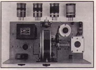
FIG. 512 - THE TOP OF THE SUB-PANEL
