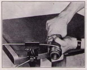
FIG. 706 — WINDING A COPPER-TUBING INDUCTANCE One and of the tubing is held in the vise and the other is flattened out and bolted to the pipe used as a winding form. Pulling on the tubing and turning the pipe in the hands, the operator walks towards the vise. The turns should be wound as closely together as possible and spaced later.
