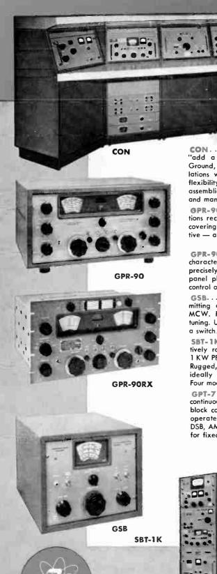
**GPR-90** (R-825 /URR) . . . a general purpose communications receiver of the double conversion superheterodyne type covering the frequency range of .54 to 31 mcs. Stable — selective — accurate — built-in crystal calibrator.
