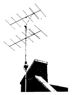
A stacked array for 144 Mc. (W1AW) which uses 5%wavelength spacing. The phasing lines and the ½-wavelength balun are joined in a weatherproof box. Element lengths for such an array can be taken from table 18-1. Element spacing is 0.2 wavelength.
