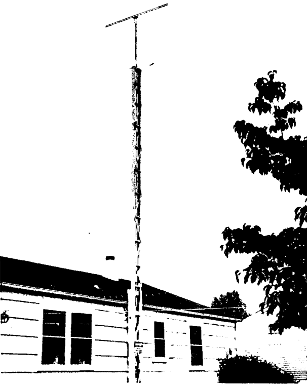
Fig. 21-57 — While guys are not normally required for the homemade tower, they provide an extra measure of protection against high winds. An inverted V can serve here as two of the guy lines.
