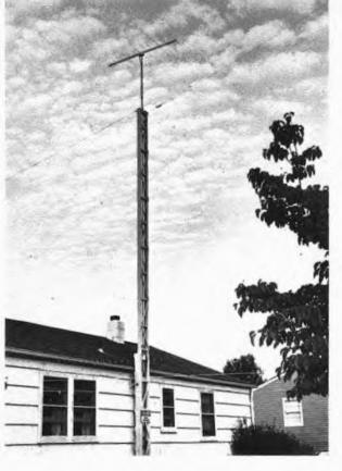
Fig. 3 — While guys are not normally required for the homemade tower, they provide an extra measure of protection against high winds. An inverted V can serve here as two of the guy lines.
