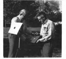
Fig. 19-2 - W1HDQ and W1\$L look for sunspots with a simple projection system. The baffle at the top end of the small telescope provides a shaded area for viewing the sun's image (light circle) on the projection surface. Sunspots large enough to affect radio propagation are easily seen with this viewing system.
