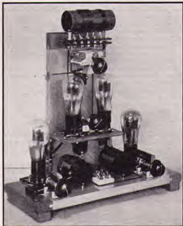
FIG. 720 — A LOW-POWER CRYSTAL-CONTROLLED TRANSMITTER FOR OPERATION IN THREE AMATEUR BANDS
