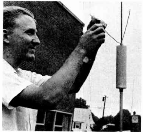
Fig. 19-36—K1MET prunes a capacity hat for antenna resonance at the low end of the 160-meter band. The Webster Big-K antenna is first tuned for the high segment of the band. The capacity hat is clipped on when operation on the "low end" is desired. Fine adjustments can be made by increasing or decreasing the spacing between the two No. 10 wires.
