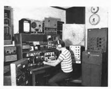
This station, owned by the Talcott Mountain UHF Society, WA1IOX, is designed expressly for moonbounce and advanced amateur satellite The work operator (WA1JLD) is able to control simultaneously the several re-ceivers, "steer" the antennas, and still have access to the peripheral equipment for data recording and measurement.
