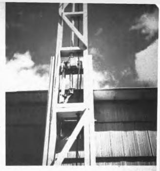
Fig. 21-59 — This close-up shows the rotor and cable installations. A double 2 X 4 is used as the base support for the rotator.
