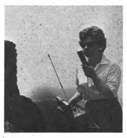
Fig. 10-1 — Effective portable operation can be realized when using lofty locations for vhf or uhf. Here, W1CKK is shown operating a battery-powered, 150-mW output, 2-meter transceiver. With only a quarter wavelength antenna it is possible to communicate with stations 25 miles or more away. Low-power transistor equipment like this unit will operate many hours from a dry-cell battery pack.
