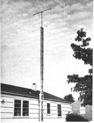
Fig. 21-57 — While guys are not normally required for the homemade tower, they provide an extra measure of protection against high winds. An inverted V can serve here as two of the guy lines.
