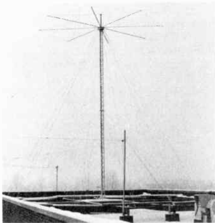
Fig. 39 — The completed discone antenna, installed on the roof of a three-story building.
