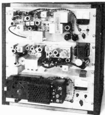
Fig. 39 — This typical 144-MHz amateur repeater uses GE Progress-Line transmitter and receiver decks. Power supplies and metering circuits have been added. The receiver located on the middle deck is a 440-MHz control receiver, also a surplus GE unit. A preamplifier, similar to that shown in Fig. 30, has been added to the 2-meter receiver to improve the sensitivity so that a 0.2\text{-}\mu\text{V} input signal will produce 20 dB of quieting.
