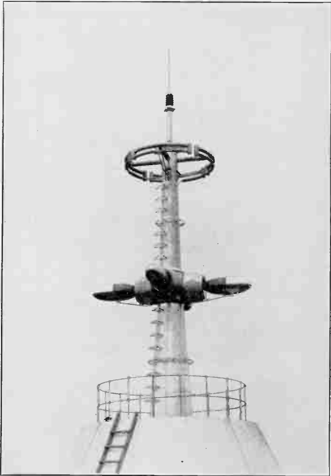
FIG. 27 —The new R.C.A.-N.B.C. television broadcast antenna as it appears on top of the Empire State Building in New York City. The antenna is located 1,200 feet or approximately one-fifth of a mile above the sidewalk of the building. The apex is a lightning rod.
