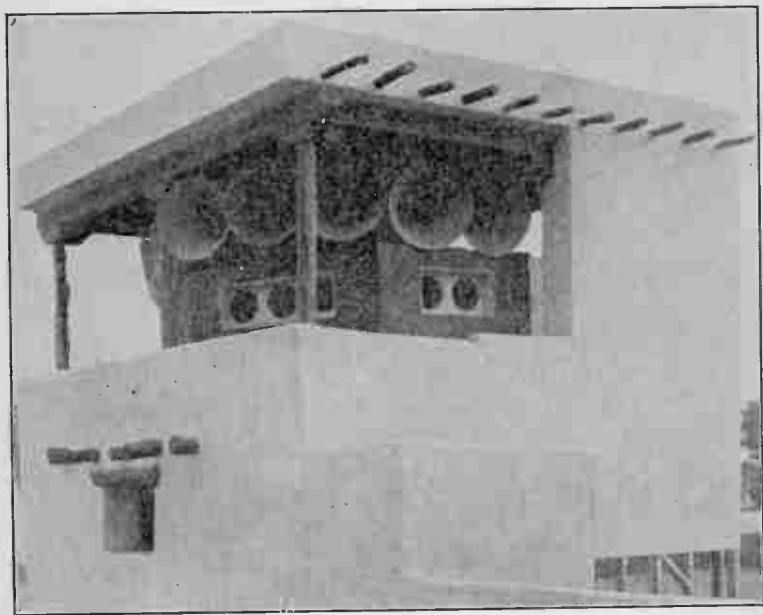
FIG. 14—Grouping of horns when used for outdoor installation.
