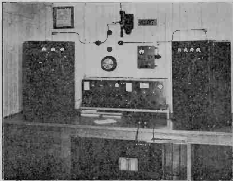
FIG. 3—Typical shipboard radio equipment installation.
