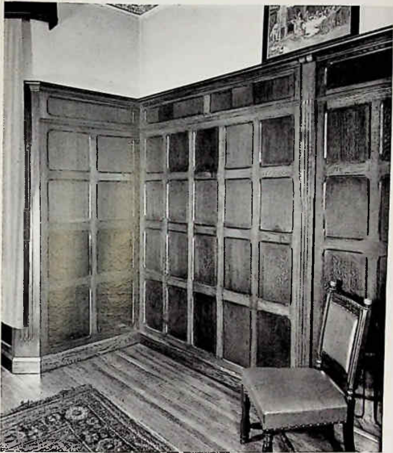
FIG. 15/6. View of panelled room which gives very good reproduction of records in spite of being square and sparsely furnished.
