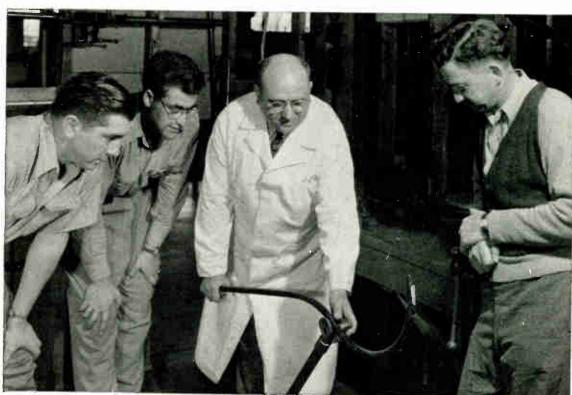
Instructor is giving a personal demonstration on handling conduit. Most of the new and modern wiring for lights and power is run in these pipes called conduit. A practical man working in this line must know how to bend, cut and thread this conduit. These Students are getting a practical demonstration on bending conduit. This training is designed to prepare graduates for work in wiring of houses, buildings, etc.
