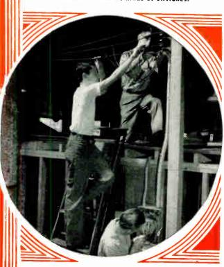
ese students are checking the installation af a modern Three-Wire Service and Service Switch, such as is commonly used in wiring homes and other buildings for lights.
