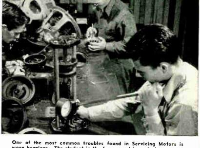
One of the most common troubles found in Servicing Motors is worn bearings. The student in the foreground is replacing a worn bearing by means of a Hydraulic Press. The students in the background are making Fractional H. P. Motor Tests.
