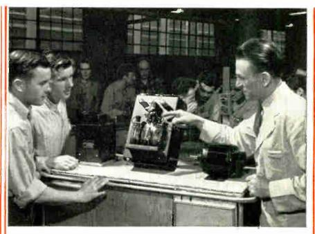
This picture shows students getting an explanation of the operation of the Thy-mo-trol, a commercial electronic unit used to accurately control the speed of a Direct Current motor.
