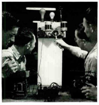
These students are building and testing Carrier Current Remote Control units, with which the power to Electrical equipment located some distance from the operator may be turned off or on by means of high frequency impulses sent aver Alternating Current power wires.
