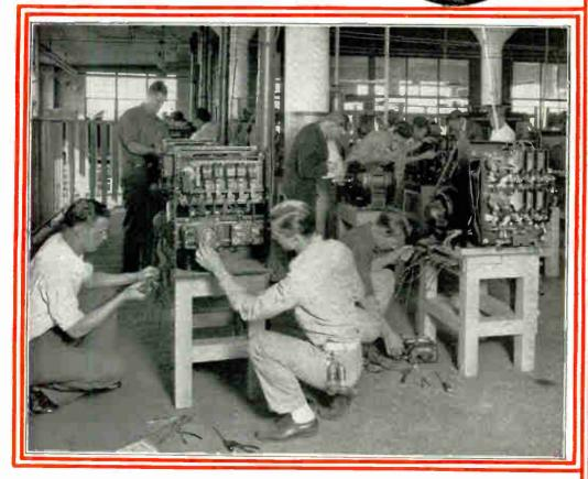
And here we have different types of modern automatic, remote control equipment for A. C. motors. These men are getting acquainted with these controls and their care and aperation, by wiring them up and testing them out with the motors.
