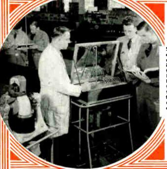
Specially designed demonstration units and personal instruction make the principles of Electricity and Magnetism clear to students. On the left is a unit for demonstrating magnetic fields around conductors and coils.
