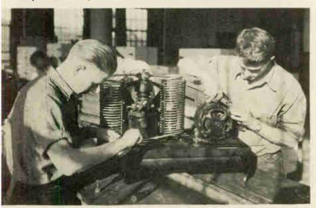
This picture, taken in our Electric Refrigeration Department, shows Coyne students carrying out the series of operations involved in the overhaul on a compressor and motor combination unit.
