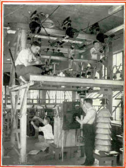
This is an outdoor type substation structure, and these students are connecting the transformers, checking the lightning arresters and voltage regulator, and becoming acquainted with this type of equipment.
