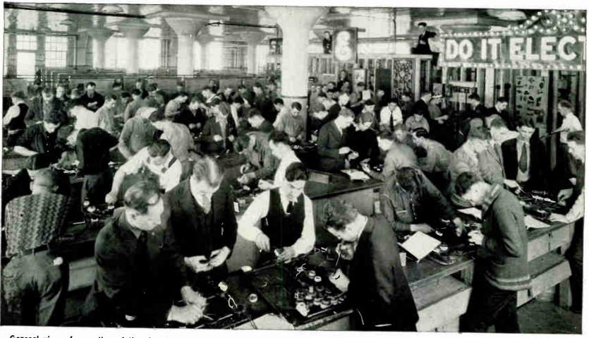
General view of a section of the electrical weining department. Notice the large and well lighted shop. The men are wiring and testing light control circuits in their first small conduit layout, and getting real practical experience in the handling of tools and the use of various kinds of switches. the use of various kinds of switches.
