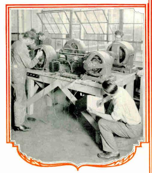
These students are operating and testing motor generator sets and measuring the output of these units.
