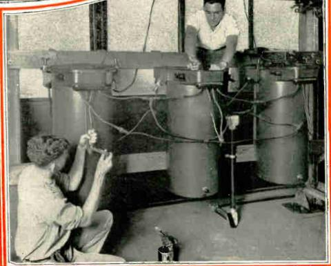
These students are connecting up a bank of power transformers for 3 phase operation, in the outdoor type substation in this department.
