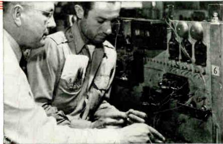
This is a close up view of a Circuit Wiring bench showing an Instructor giving a new student personal help in working out a relay circuit wiring job.
