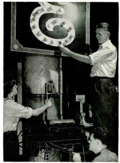
This picture shows students getting practical training in the connecting up, testing and operation of a model Electric Flasher Sign. This sign is operated by a motor driven Flasher Control which operates the "on" and "off" flasher mechanism and animates the sign.
