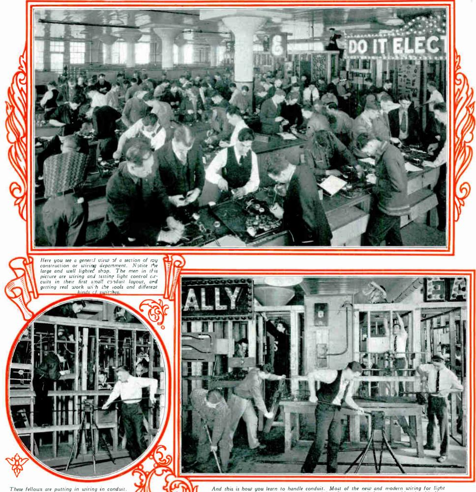
BX, and knob and tube, in the actual house frames, and learning to wire lights and switches the same as they will out on the job. And this is how you learn to handle conduit. Most of the new and modern wiring for light and power is run in these pipes called conduit. And a practical man working in this line. must know how to bend, cut and thread this conduit. These men are getting actual work with toe threading dies, hending "hickeys." and in cutting pipe.
