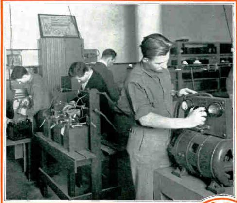
Operating a motor generator rapid charging machine, and testing batteries with a high rate discharge outfit. These are all very valuable jobs to qualify my students for the best jobs, or a business of their own. And these fellows are metting lead in a modern electric matting pot, and maulding lead posts and straps for the batteries they are building. This work gives them excellent 'practice with 'ools, and modern equipment.
