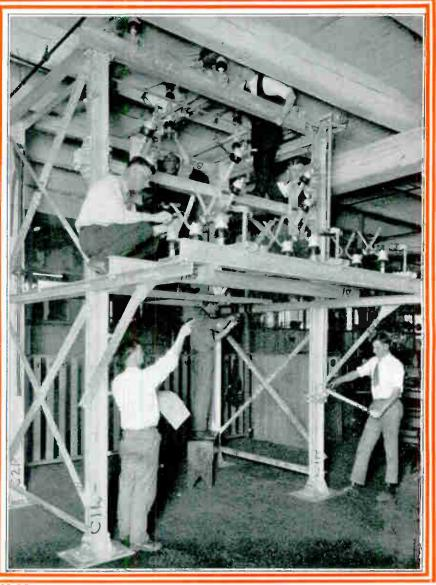
Twis is an outdoor type substation structure, and these fellows are operating the high tension switches and observing the fuses, choke coils and lightning arresters, and getting thoroughly acquainted with this kind of equipment and its construction and operation.
