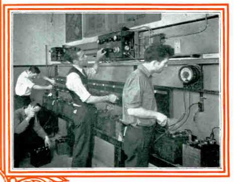
And here they are operating the charging line and equipment of the Tungar type. Both the half wave and later type full wave chargers are used here. And you see these men testing the acid, and the voltage to determine the exact condition of the batteries being charged.
