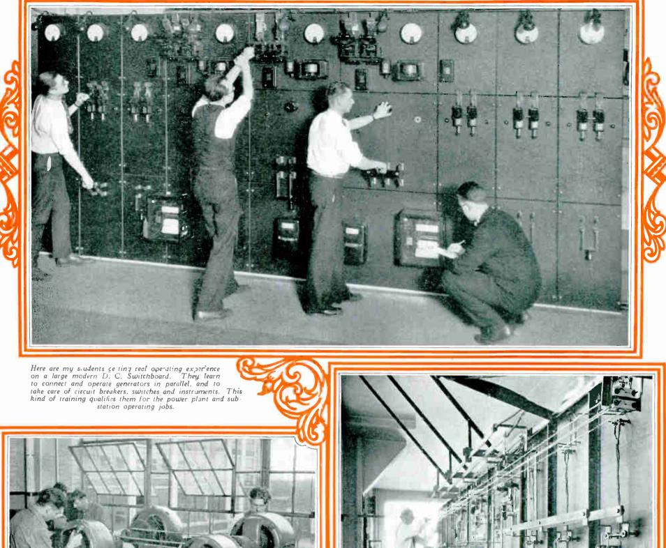
These fellows are operating and testing motor generator sets, building up voltage, and measuring output of these machines.
