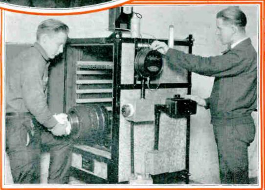
These fellows are operating the electric bake oven, and just removing an armatume that has been wound, covered with insulating compound and baked, as all armatures must be. This treatment keeps out the moisture, oil and dirt that would otherwise ruin the winding.
