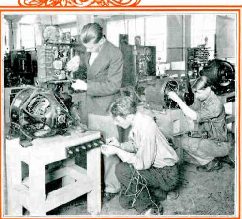
These fellows are wiring up and operating modern automatic controllers, and testing their operation right with the motors.
