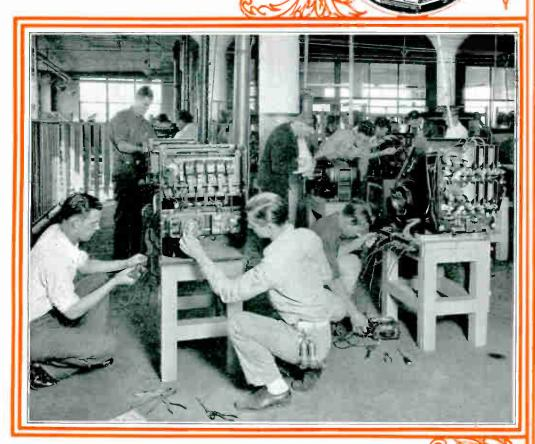
And here we have different types of modern automatic, remote control equipment for A. C. metors. These mer are getting thorougaly acquairted with every part of them and their care and operation, by wiring them up and testing them cut with the motors.
