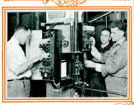
These follows are operating a carbon pile  $\mathbb{A}$ ,  $\mathbb{C}$ , motor starter, and an automatic "cross the lme" starter. A good knowledge of these devices is very important,  $\pi$ s they are widely used in many industrial plants today.
