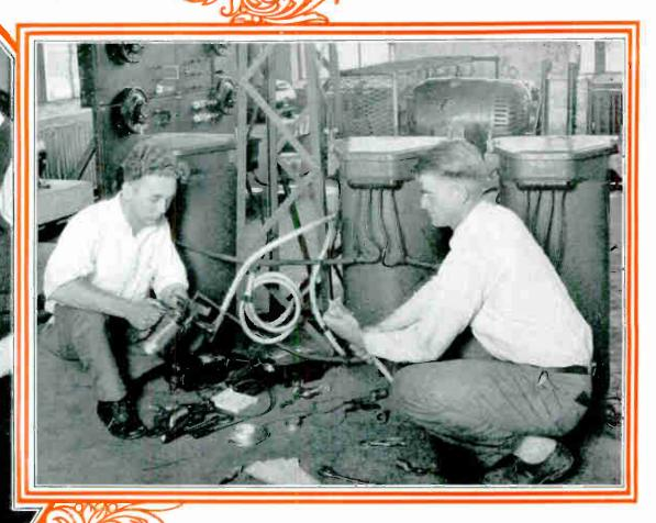
These feilows are connecting up a bank of three power transformers, and soldering the logs on the cables with a blow torch, and learning how to use the tools on the job.
