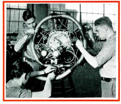
Here is where you learn the use of the twin magnetos and spark plugs for double ignition on airplane engines. And these men are also learning carburetor and value adjustment, which of course, are necessary for the proper "tuning" of the motor. There is a great and growing demand for expert ground men to work at the hangars and landing fields, and keep these motors in "tune."
