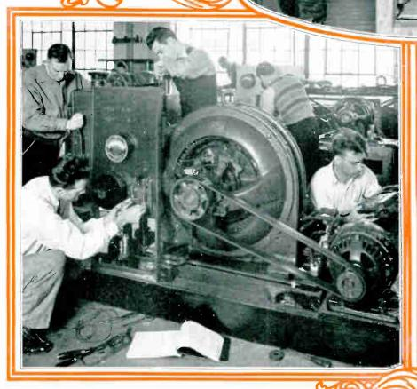
Here you see several of my students commeting, testing, and operating a large synchronous motor, and its exciter generator. This machine is also used for correcting power factor, and every up-to-date, well trained man should know this work well, to qualify for the best jobs.
