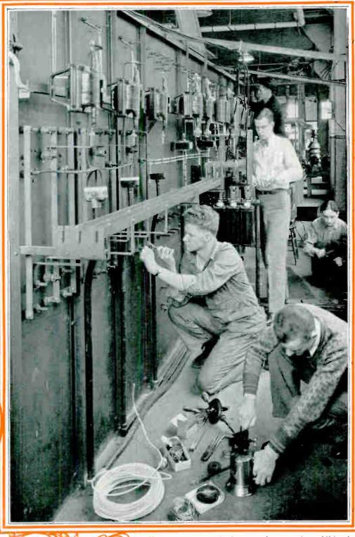
Here you see severa, If my studen 3 putting additional circuits on the main A. C. switchboard. They are installing bus bars, cables and conduit, and instrument transformers. So you see how my complete training qualifies you for anything that comes up on the job.
