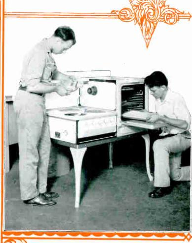
My shops are kept up-to-date. Here is an electric range, with automatiz temperature control equipment. These fellows are learning how it is constructed, and wired, and where to look for any troubles that might develop in such equipment. In many localities where hydro power makes electricity lower in cost, these electric ranges are being sold and installed by the thousands, creating gocc jobs for trained men to wire and repair them.
