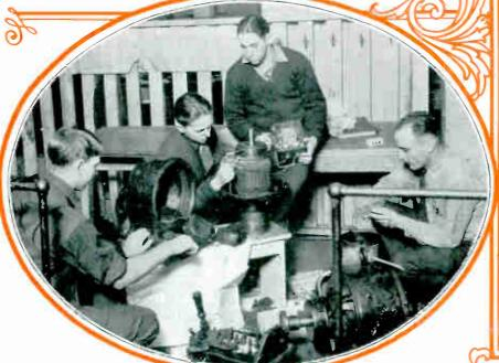
Here is another complete overhaul and repair job on a motor generator. These men are testing the armature with a magneto, and repairing the field coils and brushes.
