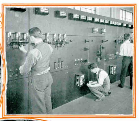
And these men are getting actual operating practice on a large A. C. switchboard. Here they learn the operation and care of meters, circuit breakers and switches, and how to synchronize and operate alternators in parallel and equalize their load. And in this way gualify for the fine positions in A. C. Power plant operating.
