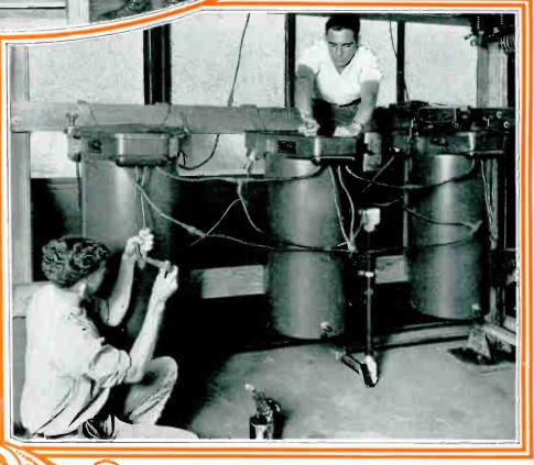
There fellows are connecting up a bank of power transformers for 3 phase operation, in the outdoor type substation in this department.
