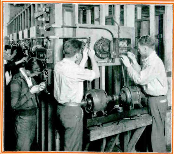
Here are some of the motors the fellows wire and test in this department. This actual work teaches them how motors and statters must be wired according to the code, and how to test to locate troubles in the wiring, which might cause motors to fail to operate. And it gives them still more practice in the use of tools. Don't you agree that to "Learn by Doing" is certainly best?
