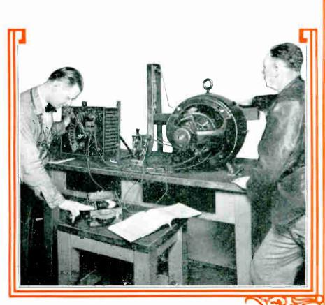
And this is a horsepower test, you earn to test the horse-power and efficiency of motors, and to select the proper motor for various jobs they are used on
