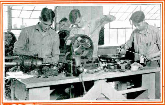
Real practical training. These fellows are completely overhauling and repairing a D. C. motor, and repairing the field coils, and the commutator and armature.
