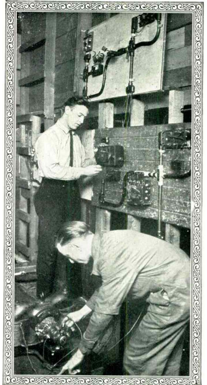
Motor Wiring and Installation
