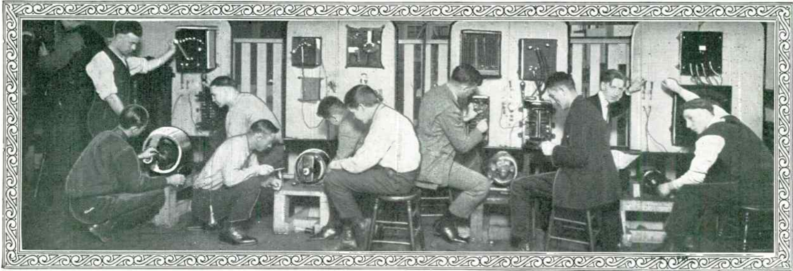
Students Wiring Up and Operating Various Types of D. C. Control Apparatus and Motors
