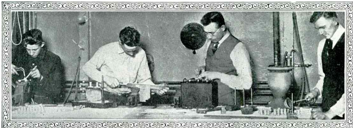
Students Acquiring Speed in Battery Repairs. Tearing Down and Rebuilding a Modern 3-Cell, 6-80 Battery
