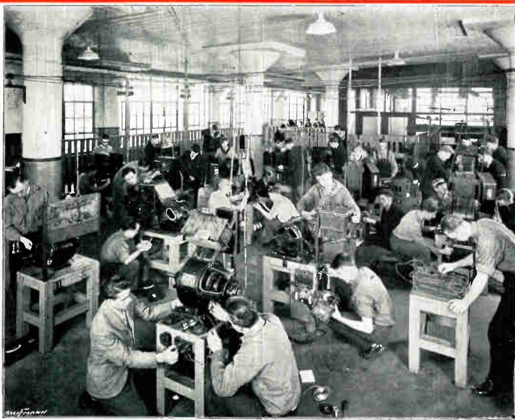
These fellows are connecting up, testing and repairing various types of A. C. motors and controls. When they understand their operation, use, and care, the instructor checks their work, so they know it is right, and when they leave school to take a job on the outside, it seems just like changing from one job to another.
