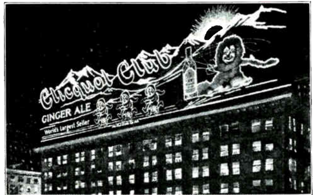
Fig. 208. Large signs of the above type often use several flashers, and a combination of lamps and Neon tubes to produce very beautiful effects.
