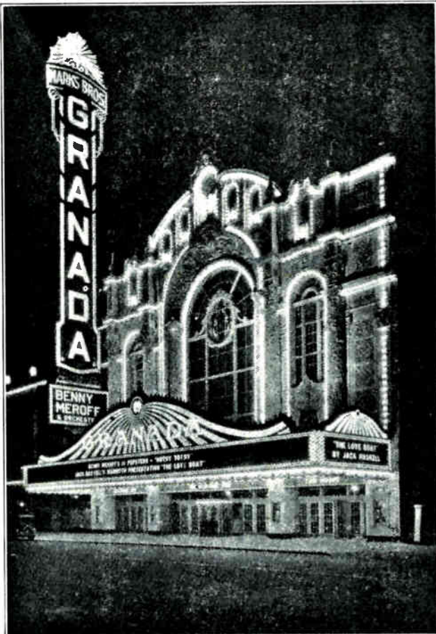
Fig. 211. This photo of the front of a large theatre shows what beautiful effects can be obtained by the use of flasher signs and lights on the building itself.
