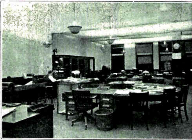
Fig. 193. This office is lighted with indirect units which are ideal for avoiding all glare and shadow effects. (Photo Courtesy Light Magazine).
