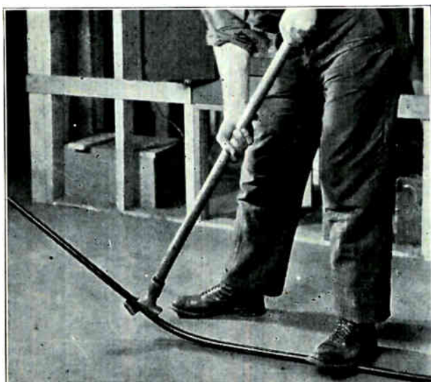
Fig. 63. Smaller sizes of conduit can be easily bent into the required curves and shapes with a bending "hickey", in the manner shown here.
