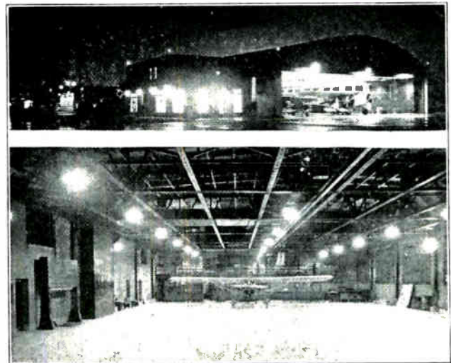
Fig. 233. The top view shows the outside appearance of a well lighted hangar, and below is shown the inside of the hangar and the arrangement of the lighting units.
