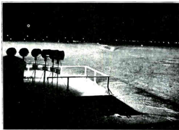
Fig. 227. This landing field is lighted with a group of small flood lights such as shown in Fig. 225.
