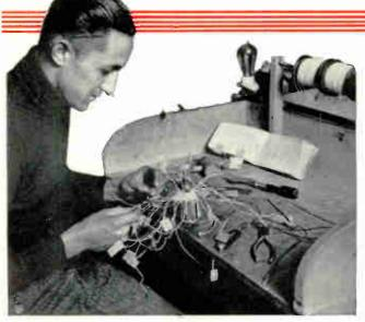
This man is testing a finished winding of a small D. C. armature, before connecting the leads to the commutator. These actual wire windings you do first on these small armatures get you acquainted with the use of tools and handling of coils, so you are ready for the large windings which come next in this department partment.
