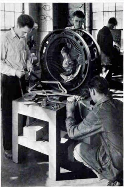
And these men are taping and putting in new coils in a 100 horsepower A. C. stator. This is the kind of actual work that fits a fellow to handle a job in the field. And when you have done actual work like this you have the ability and confidence to tackle repair jobs.
