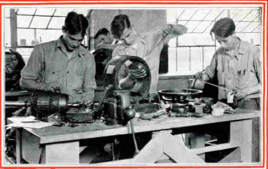
Real practical training. These students are completely overhauling and repairing a D. C. motor, and repairing the field coils, and the commutator and armature. The armature can be called the heart of D. C. motors. These naturally require attention from time to time.
