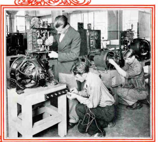
These students are wiring up and operating automatic controllers, and testing their operation right with the motors-
