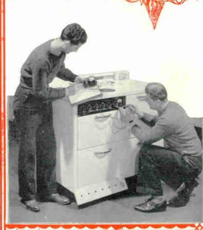
Here is an electric range, with automatic temperature control equipment. These students are learning how it is constructed, and wired, and where to look for any troubles that might develop in such equipment. In many localities where hydro-power makes electricity lower in cost, these electric ranges are being sold and installed by the thousands, creating jobs for trained men to wire and repair them.
