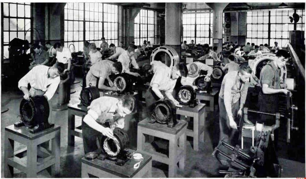
Here you see a view of part of the Stator Winding equipment. Notice the large, airy, and well-lighted shop these men are working in. Actual winding and testing of Alternating Current motors of various sizes gives you the practical training you need in this work. Motor repair work of this kind is often necessary in Electrical maintenance jobs in Power Plants, factories stores, office buildings and, in fact, wherever Alternating Current motors are used.
