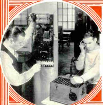
These men on the left are wiring and testing telephones. The instructor explains the operation of each part and then the students wire up the phones and test out their work by talking over them.
