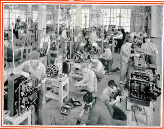
Another view of a section of our A. C. department showing students working on a wide variety of A. C. motors and control equipment. You learn how to inspect, connect up, test and repair many types of A. C. machines. This practical training in modern maintenance work makes a fellow more valuable to his employer.
