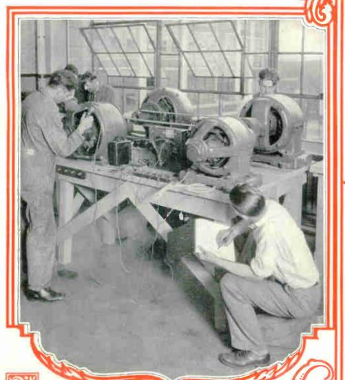
These students are operating and testing motor generator sets, building up voltage, and measuring the output of these units.
