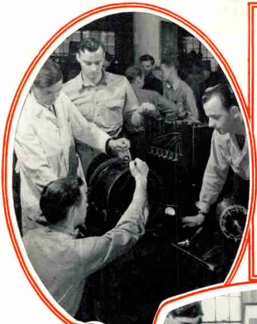
Real practical work overhauling and repairing an A. C. induction motor. When you understand the working parts of such equipment you have confidence in your knowledge of this work.
