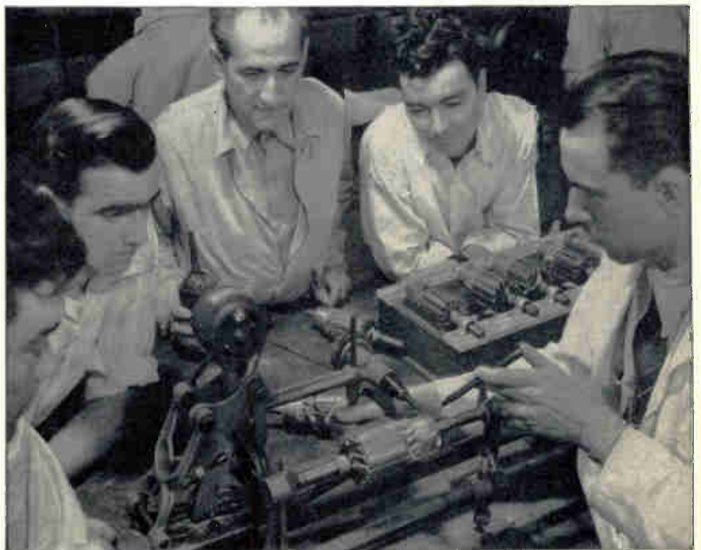
Above you see a group of students learning how to use a Commutator Undercutting Tool and the proper procedure in undercutting the mica of a Commutator. This kind of real practical training teaches them the proper use of equipment and proper methods to save time and do first class work.
