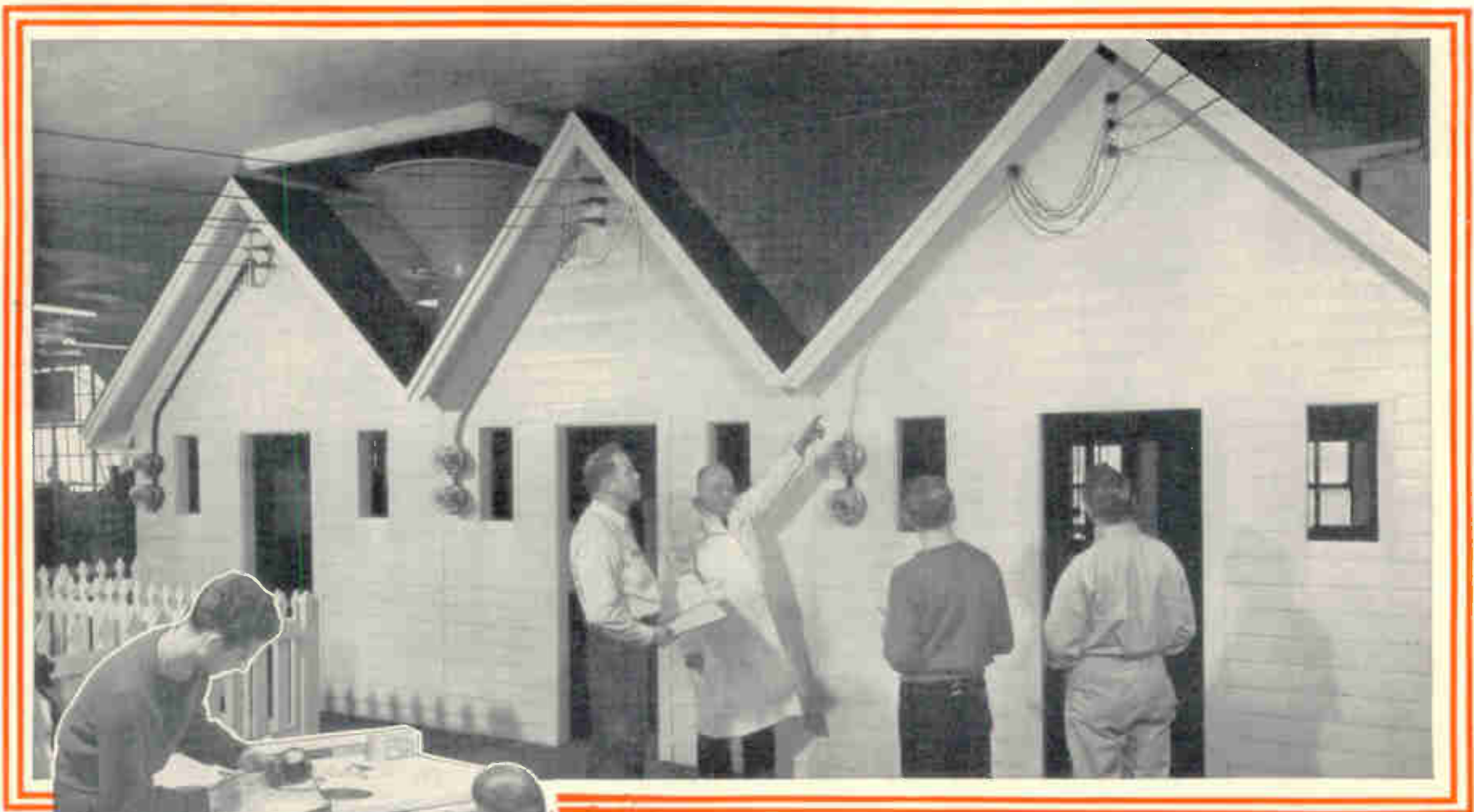
This is a picture of a Model Framework of a Bungalow which has been set up for students to get training under similar conditions as they will find out in the field. Here you see students getting instruction on the proper installation of a Service and Meter System.
