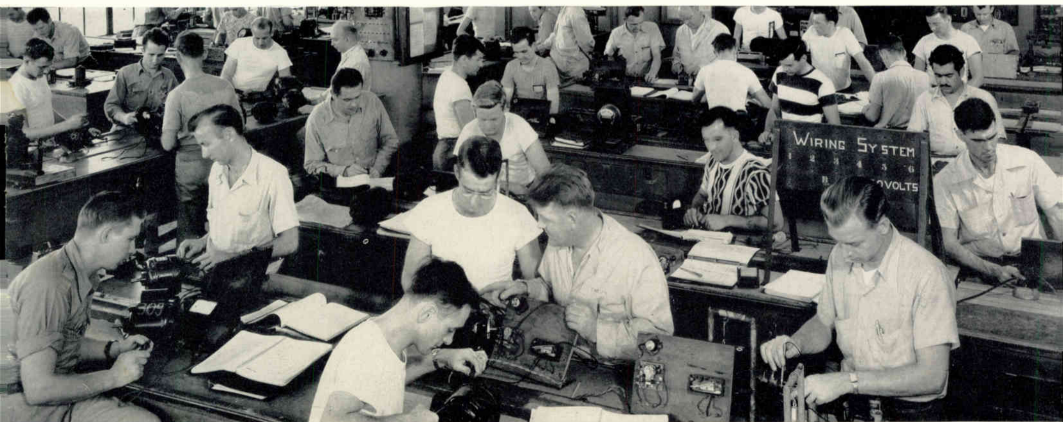
This is a general view of our Wiring and Repair Department showing students getting real practical training on various Testing, Adjusting and Repairing operations on Motors, Controls and other types of Electrical apparatus. This is a profitable field of opportunity to the trained Electrical man, whether he is working for a Service Organization or Operating a Business of his own.
