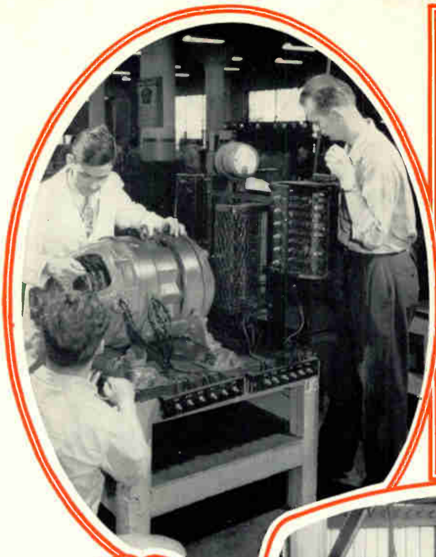
The picture above shows an instructor explaining the operation of an A.C. Motor and Control equipment with which these students are working. Actual experience on such interesting equipment is of great value to the student.
