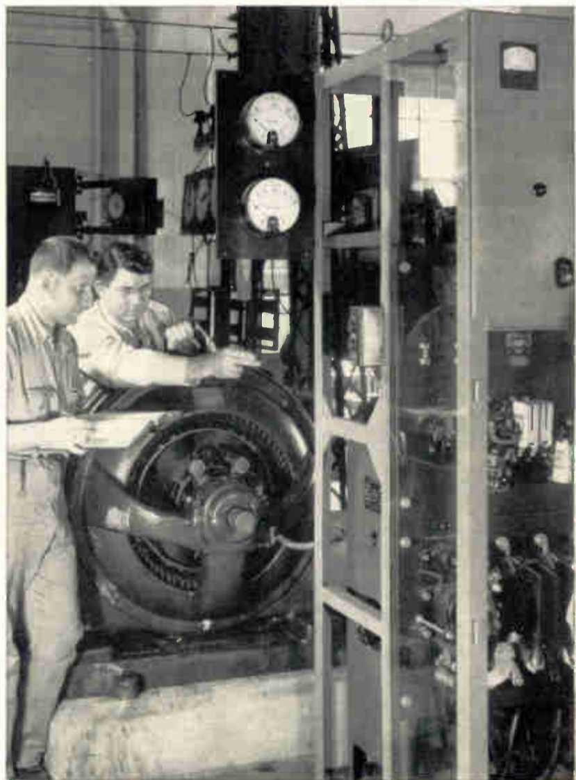
The above photo shows an Instructor explaining the operation and adjustments for synchronous type motor and students preparing to make tests. This unit is used for correcting Power Factor. Every trained maintenance man should be familiar with this type of work.
