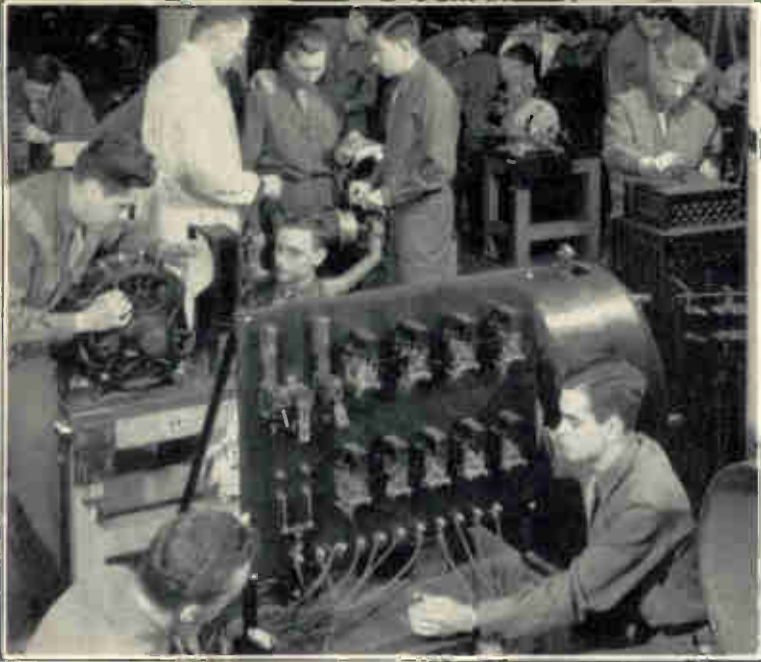
This is how our students get training on relay and control equipment, and are taught how to quickly locate trouble, so they can save time and money for their employer on the job.
