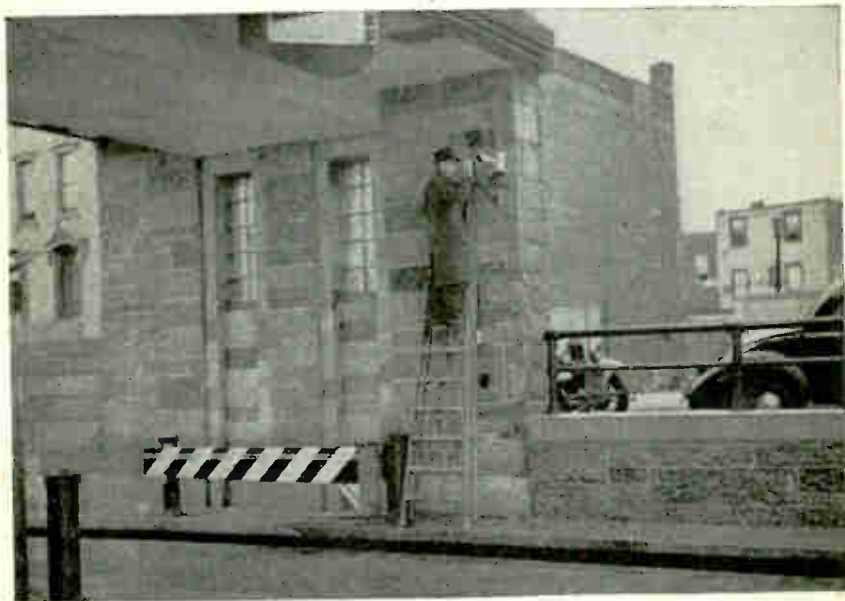
Fig. 278. A phototube-operated warning signal at a tunnel approach. A motor truck high enough to interrupt the light beam to the phototube is too high to pass through the tunnel, and the phototube causes a warning signal to be given.
